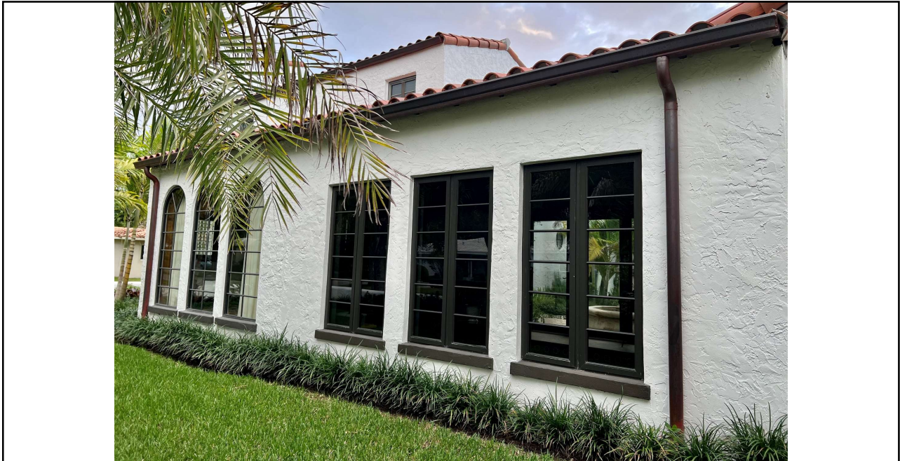
West Façade – After
