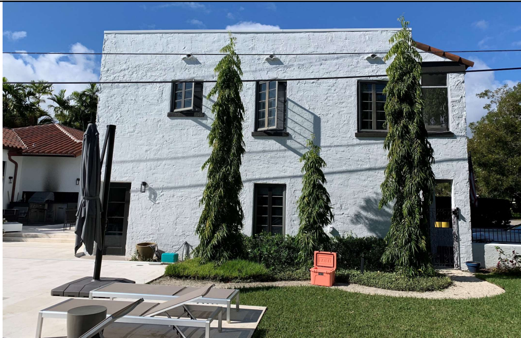
East Facade – After
