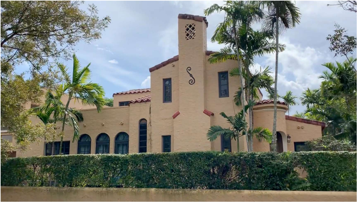
North Façade – Before
