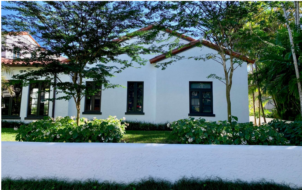
West Façade – After
