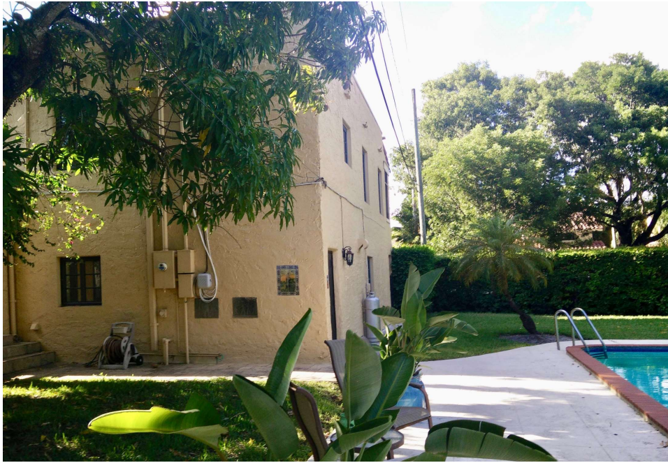
South Façade (Back of Garage) – Before
