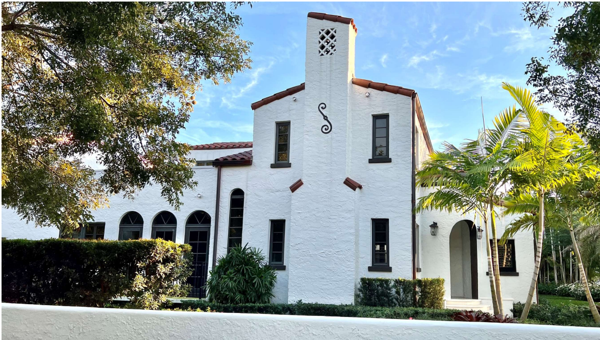
North Façade – After
