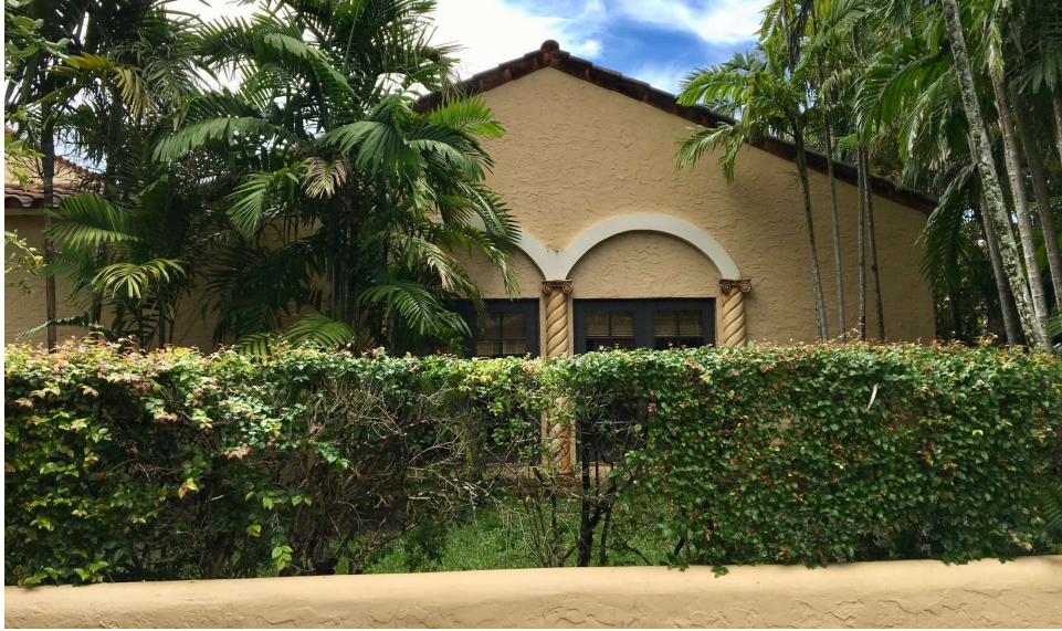
West Façade – Before
