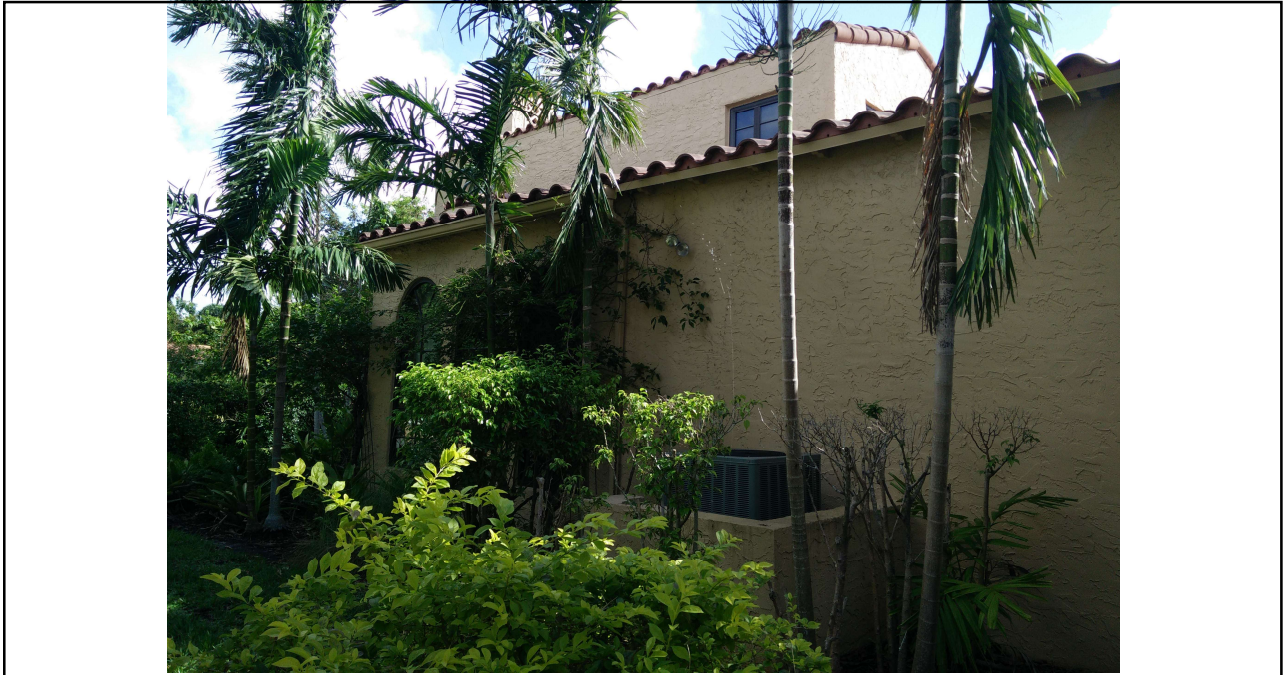
West Façade – Before
