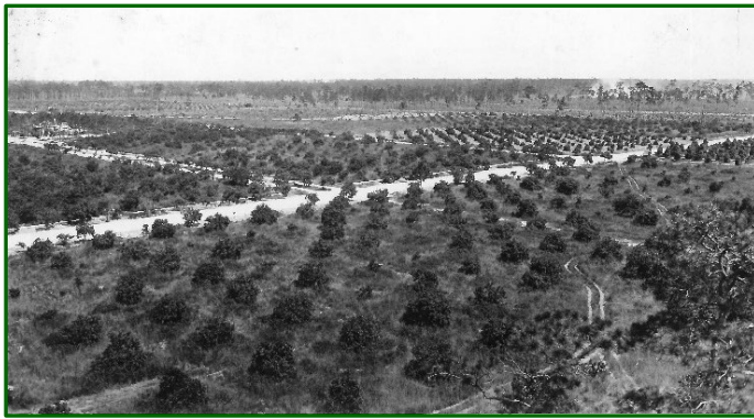
Figure 1: Streets in Coral Gables Under Construction, July 22, 1922
