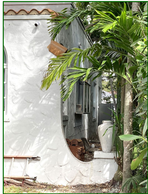
Figure 20: East Façade Looking North, 2025
