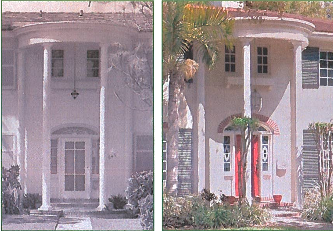
Figures 10: Front Façade, 1940 [left], Current [right] Neoclassical two-story columned round portico and front door assembly
