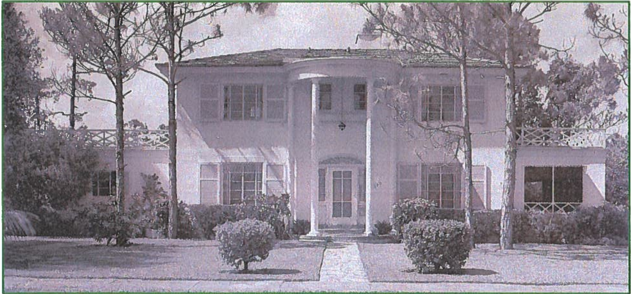
Figure 7: 649 Palmarito Court: Front (South) Façade, c.1940s
