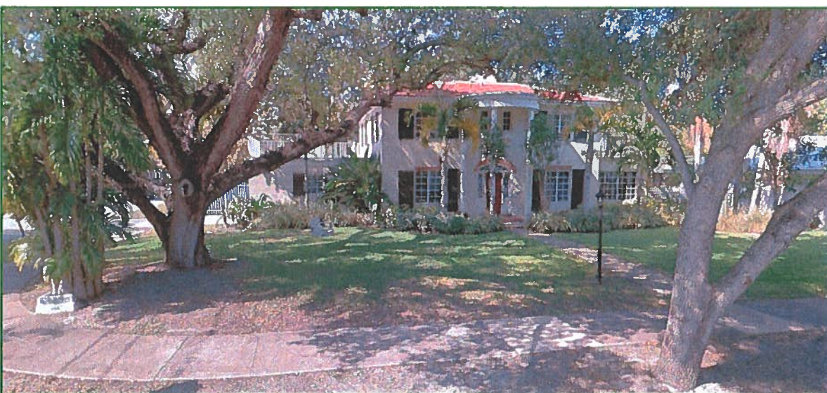
Figures 8: 649 Palmarito Court, Front (South) Facade Courtesy of Google Earth
