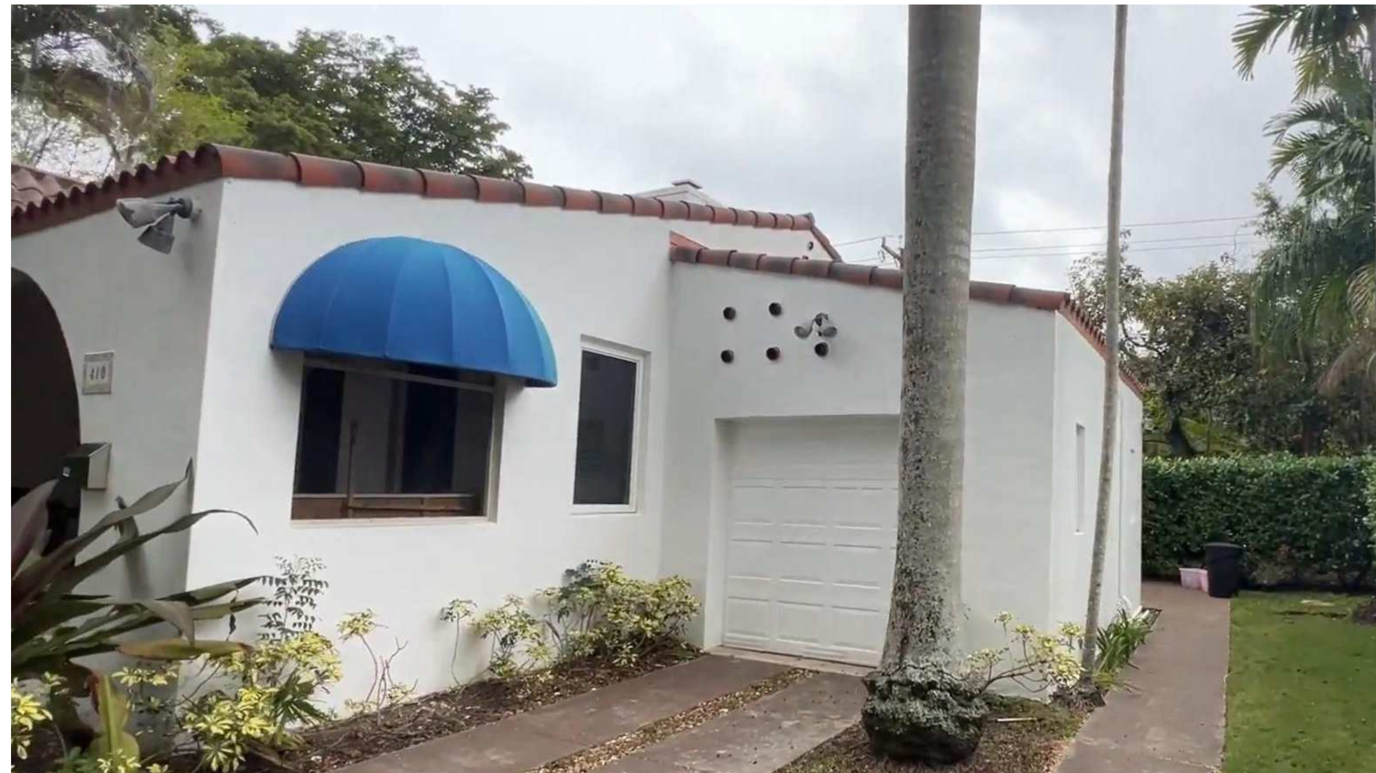
WEST, NORTHWEST, LOOKING EAST, SOUTHEAST
