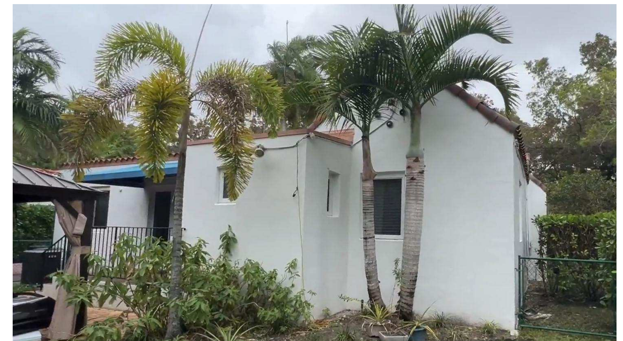
REAR VIEW LOOKING NORTH, NORTHWEST
