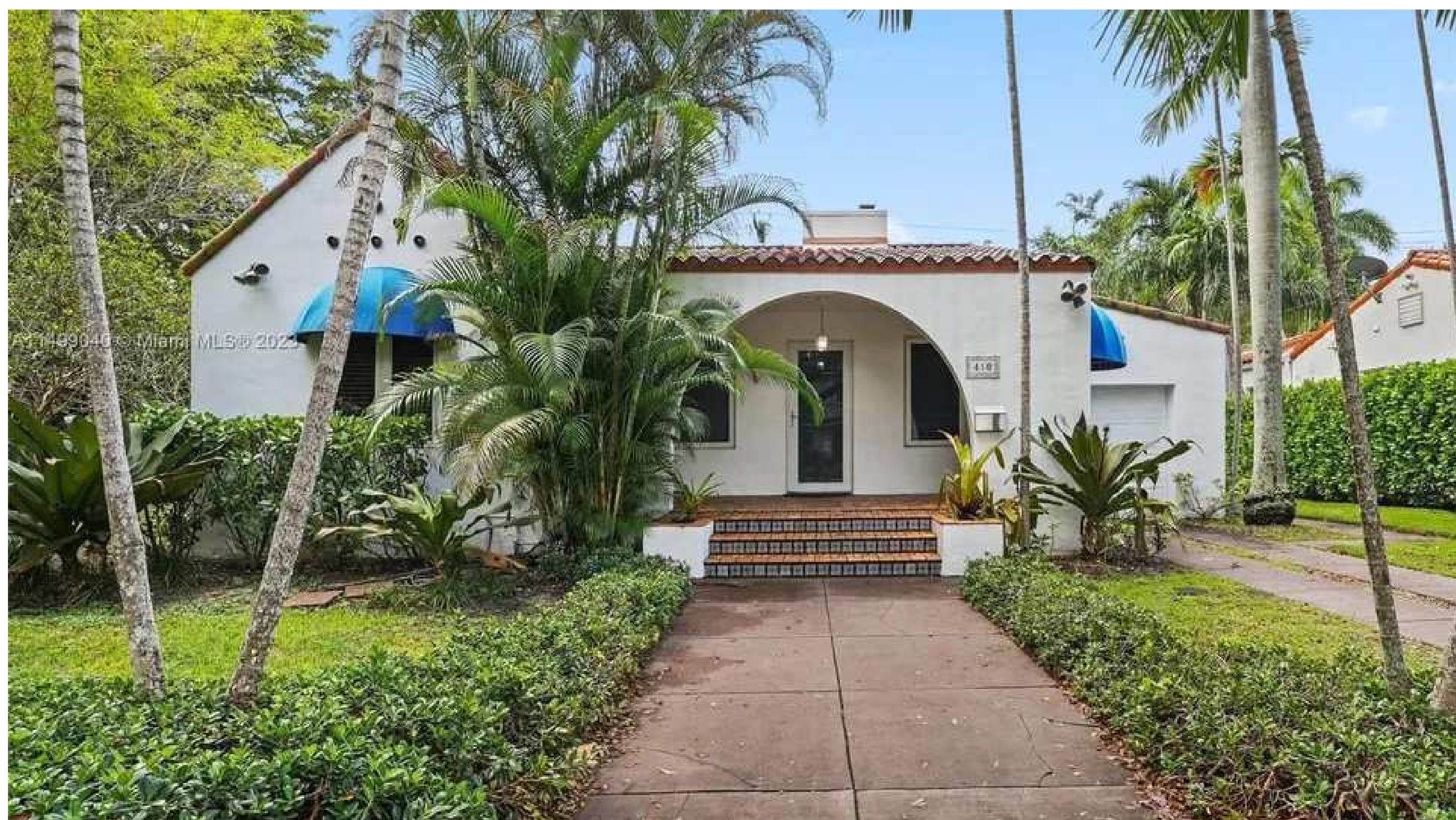
SOUTH VIEW (ENTRANCE)
