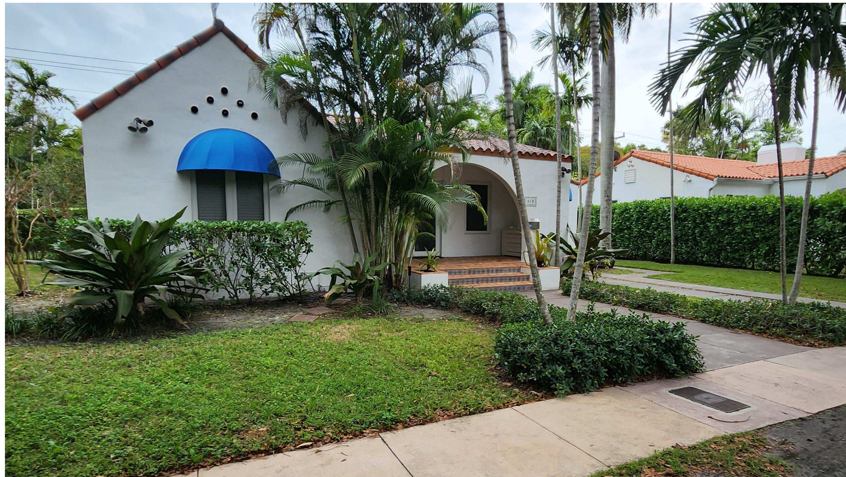
VIEW FROM STREET, LOOKING SOUTH
