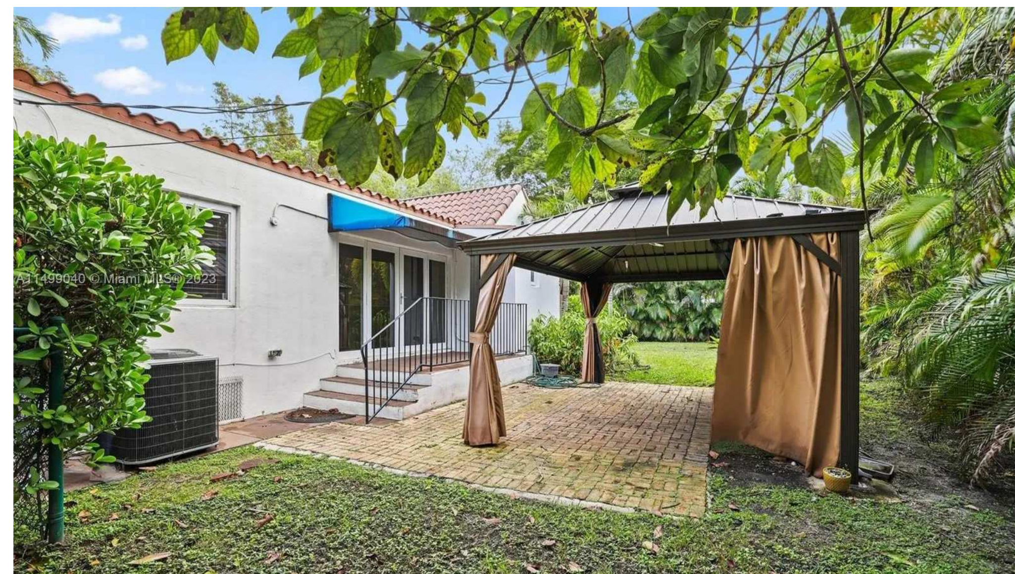
REAR VIEW LOOKING EAST, NORTHEAST
