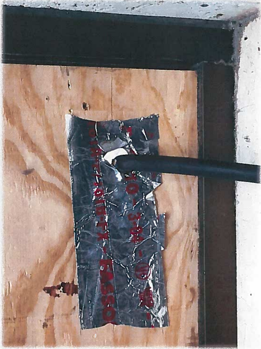
Plywood on window enabling portable air conditioner
