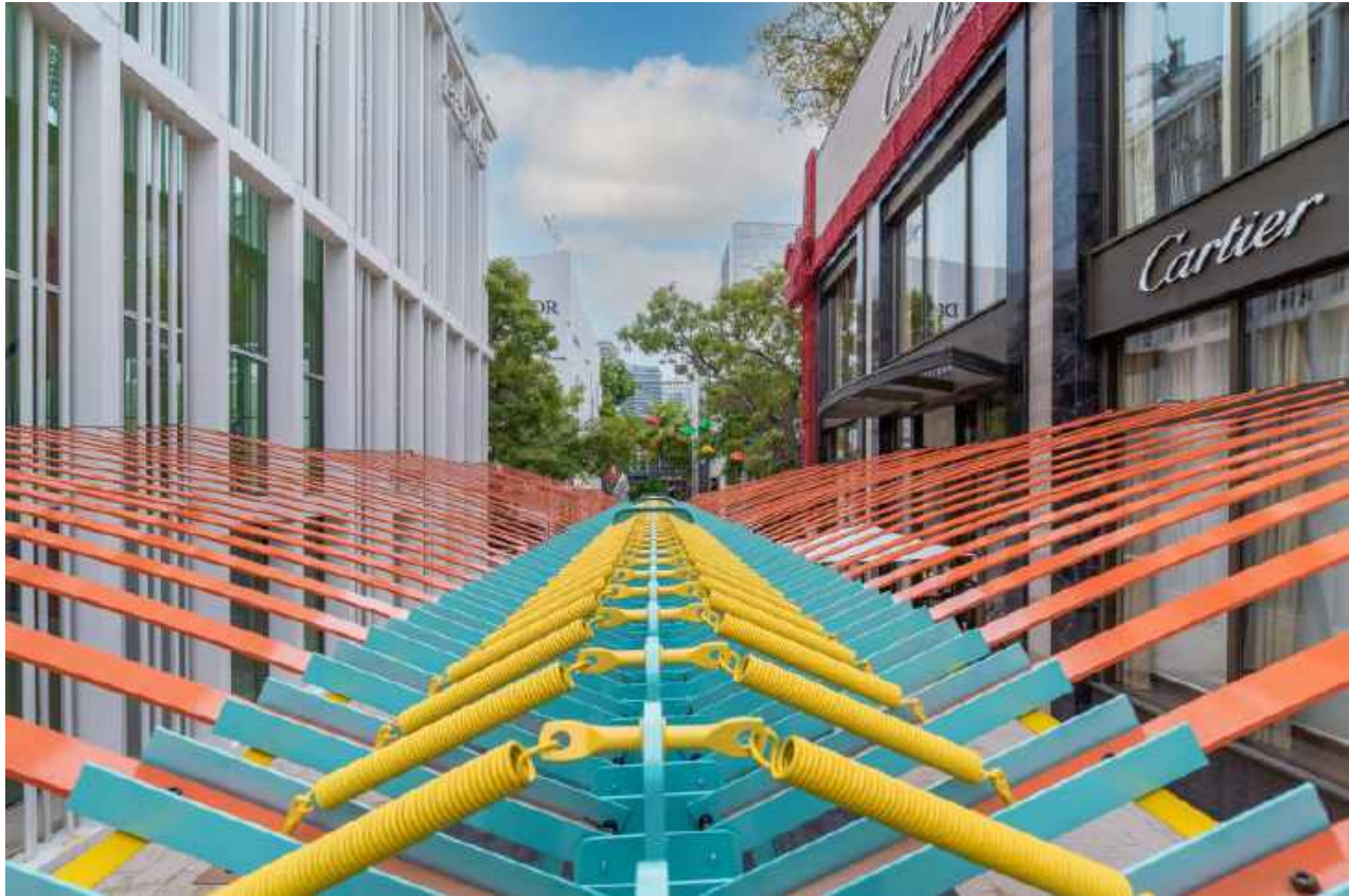
Yellow springs run along the top of the structure. Photo by Luis Gomez
