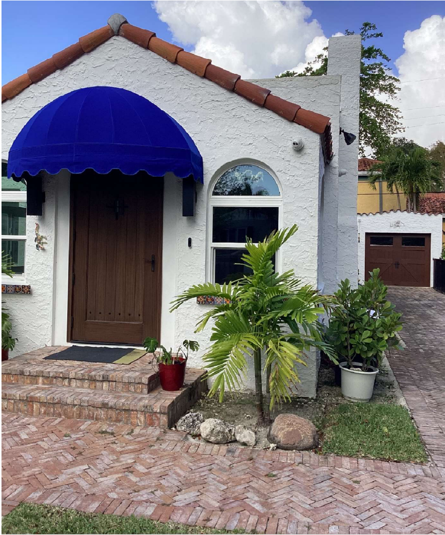
West & North Façades – After
