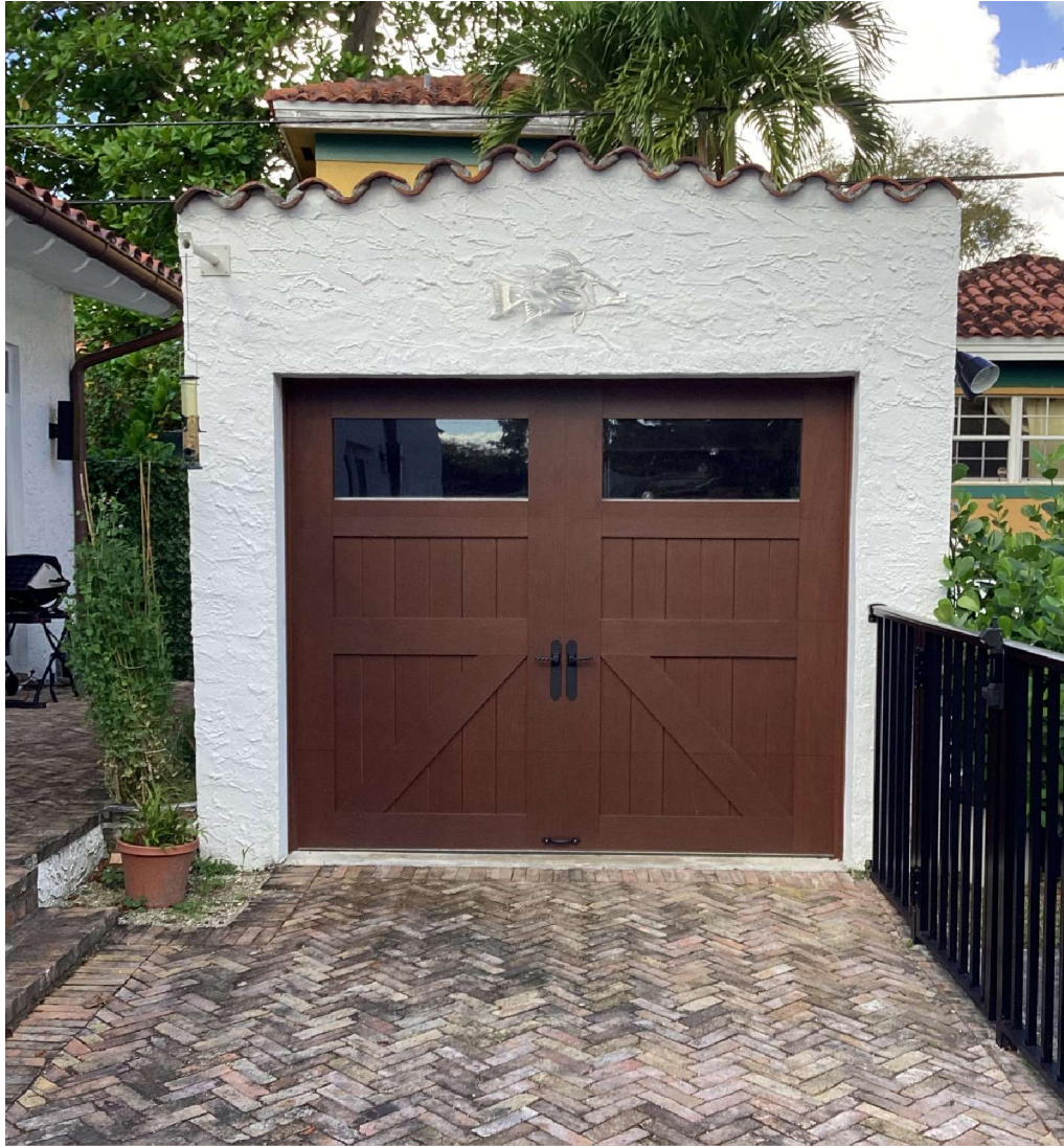
Detached Garage (East Façade) – After
