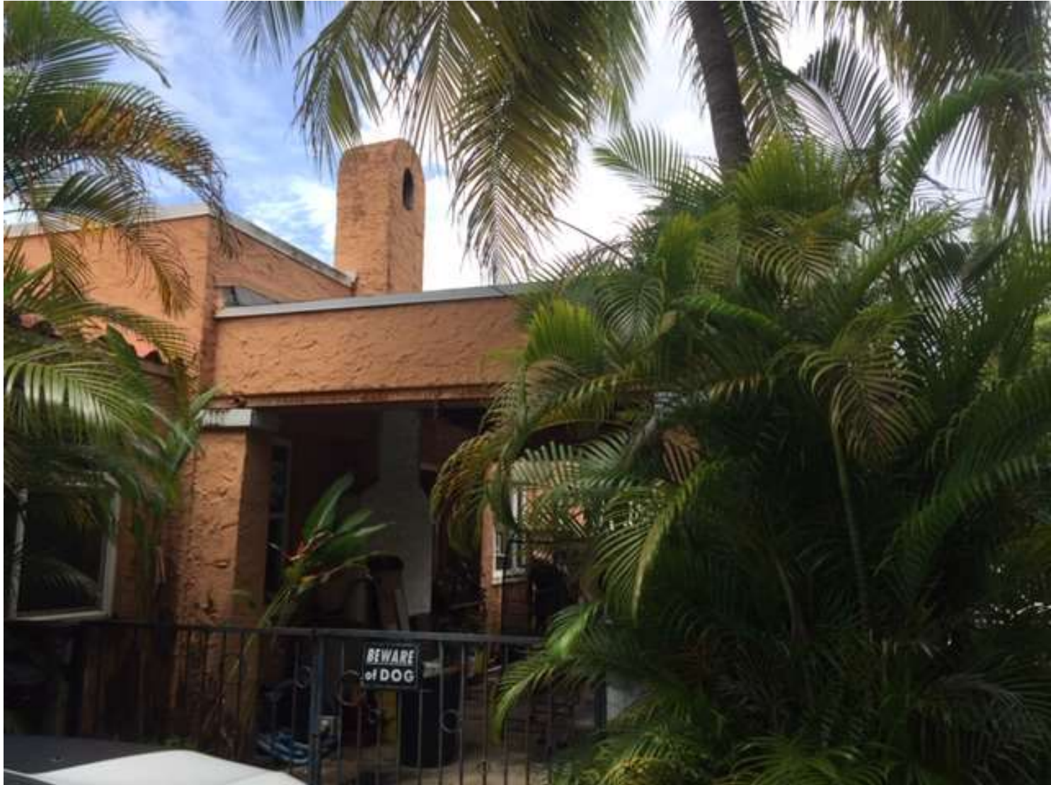
North Façade – Before
