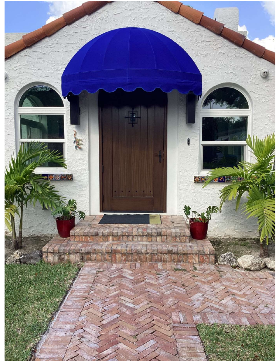
Front Entry Projecting Bay – Before & After
