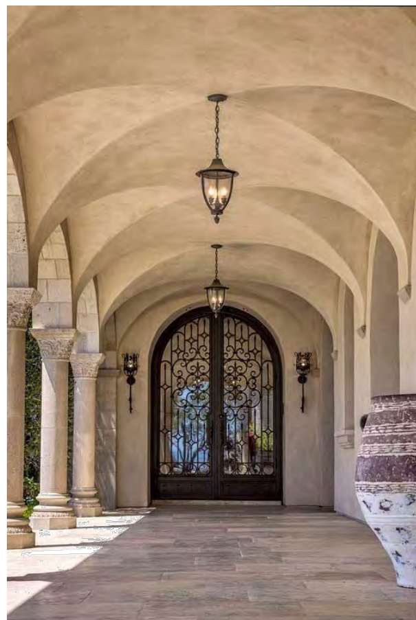
CLASSIC GROIN VAULT INSPIRATION
