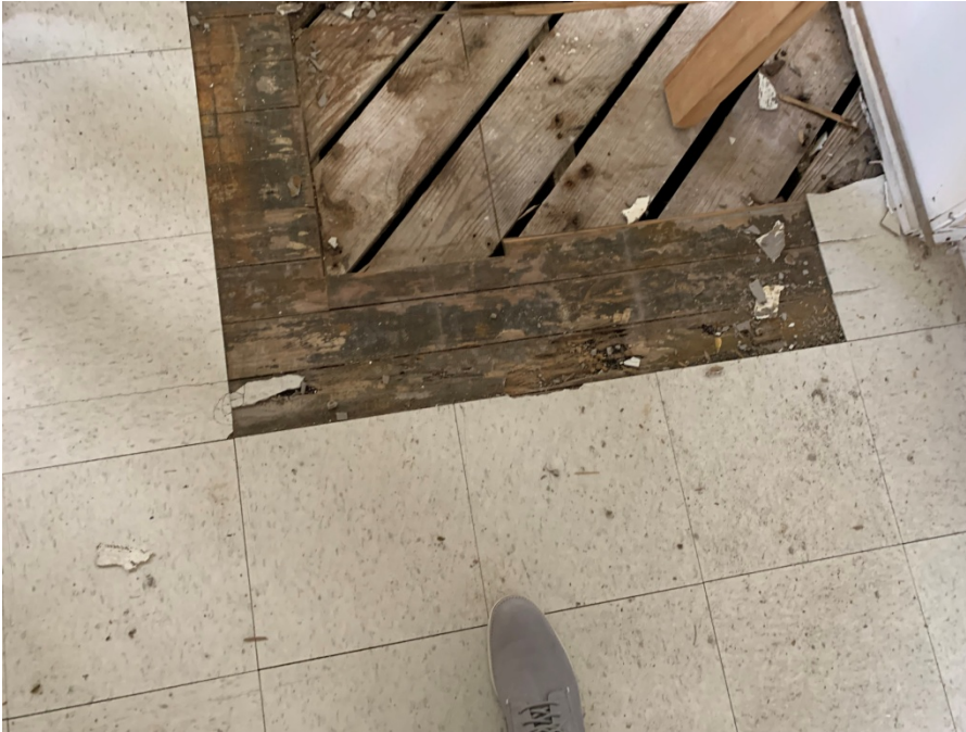
Picture #9 Wood floor damaged by termites.
