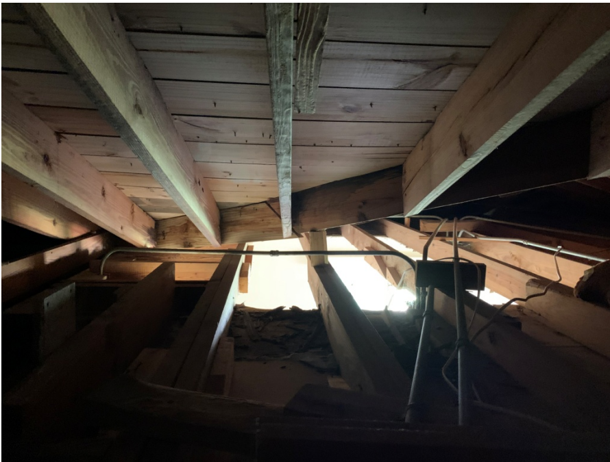
Picture #10 Ridge joist broken.
