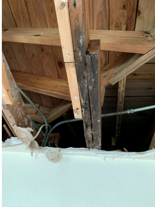
Picture 1 Area of the roof previously affected by water intrusion.
