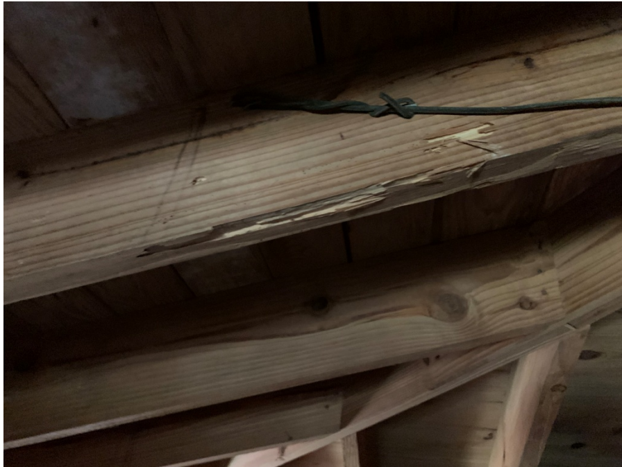
Picture 3 Roof joists damaged by termites.
