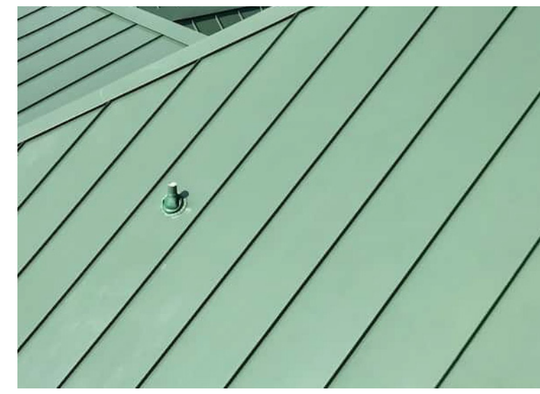
5. STANDING SEAM ROOFING (COPPER PATINA COLOR)
