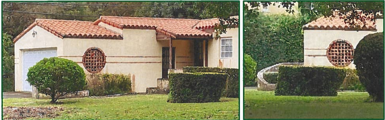
Figures 18: Northern Wing Containing the Garage, 2024
