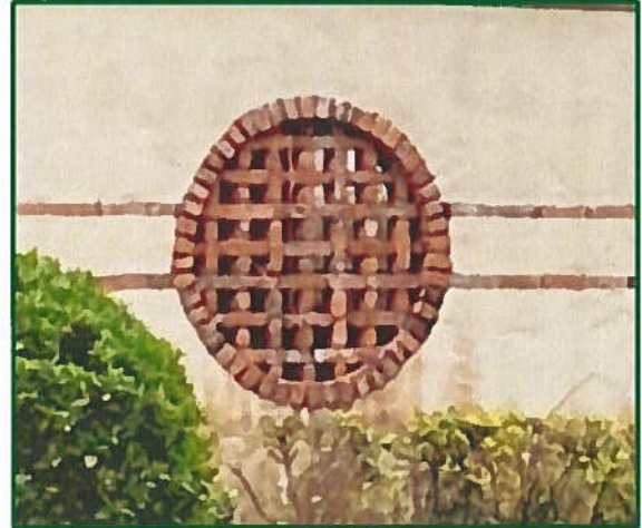
Figure 9: Garage ‘Porthole’ Brick Screen, 2024
