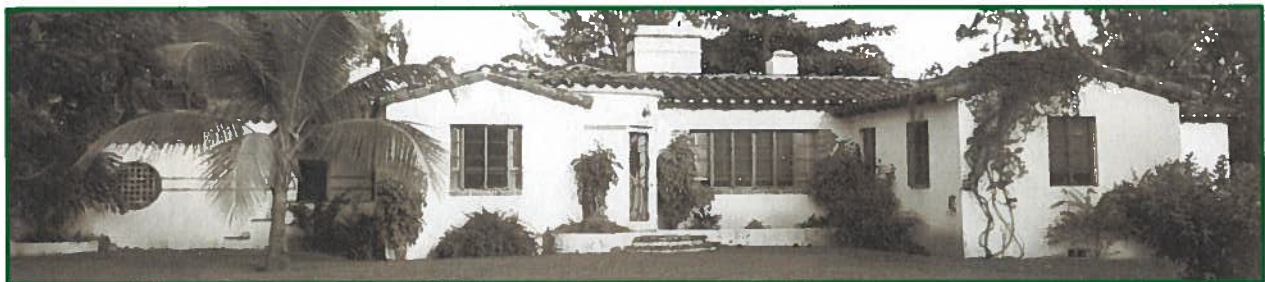
Figure 13: Front (West) Façade, c.1942
