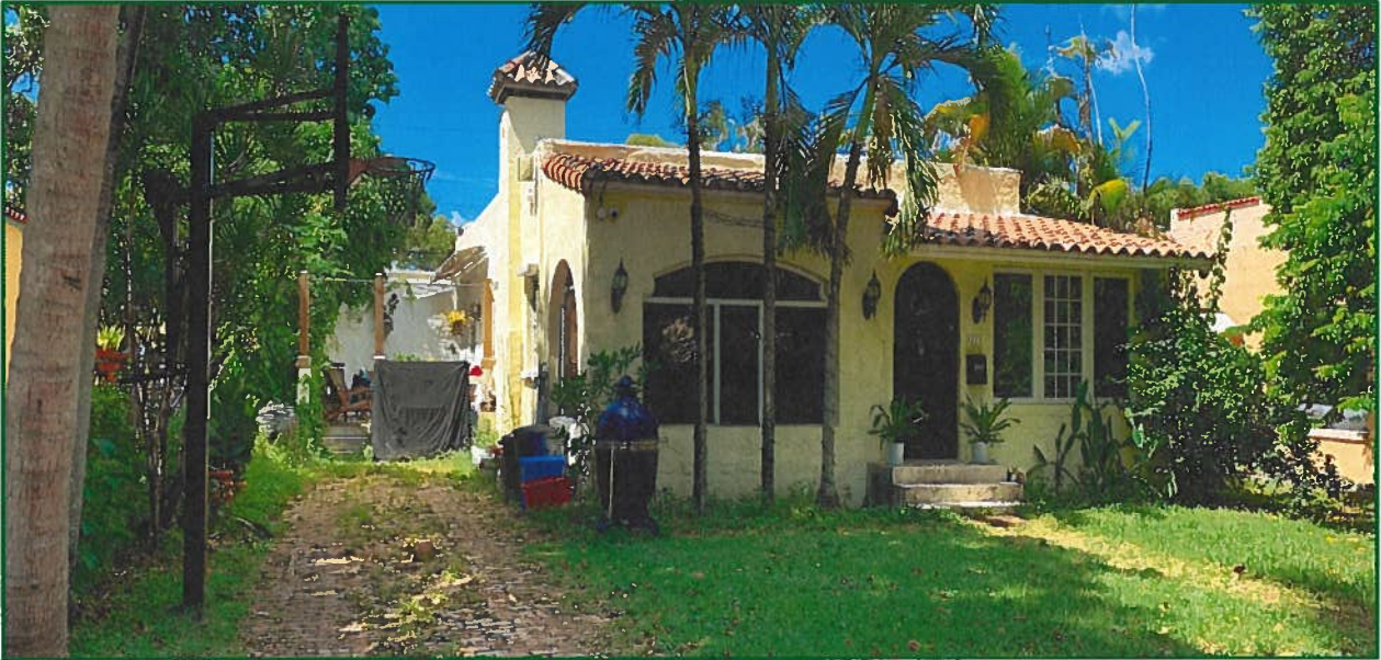
Figure 19: 1221 Milan Avenue, Front (South) Façade, 2022
