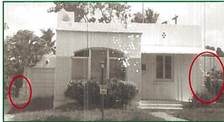
Figure 23: Historic Photo, 1967 Red circles: Wing Walls
