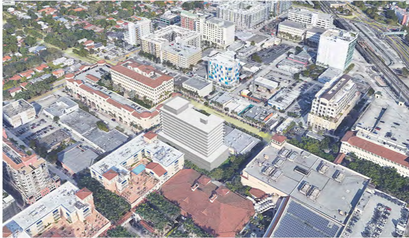
AERIAL LOOKING NORTHEAST
