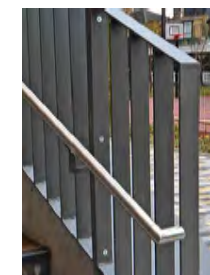
FLAT BAR HANDRAIL
