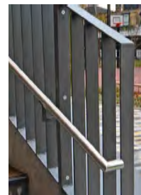
FLAT BAR HANDRAIL
