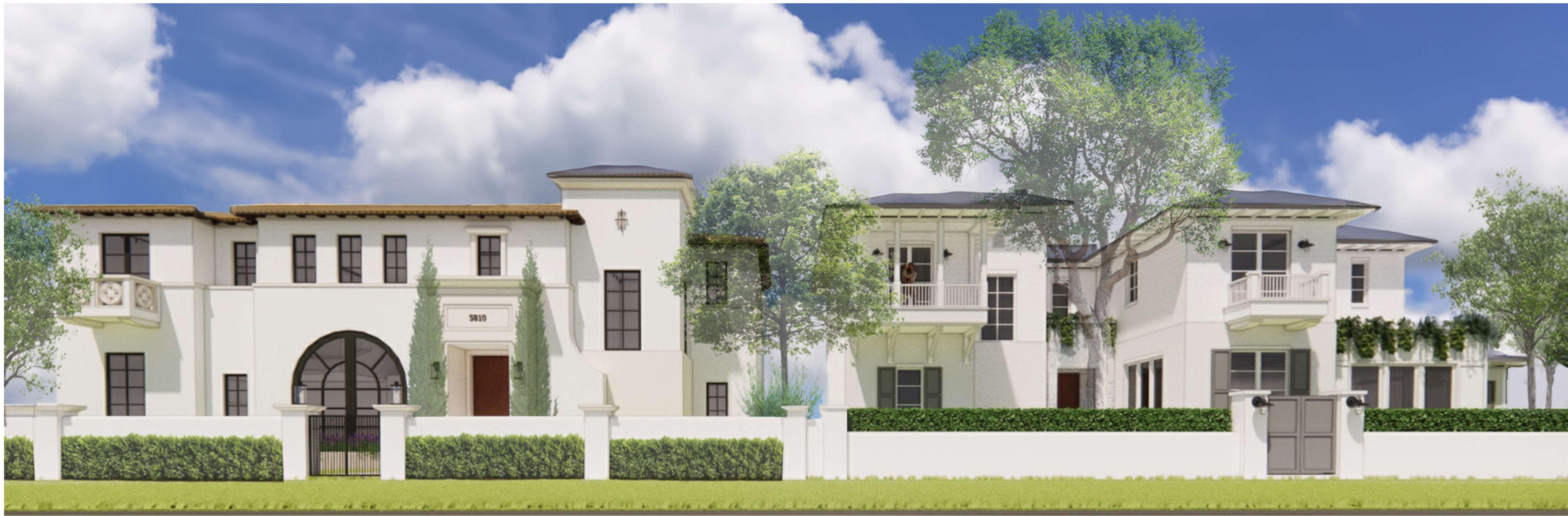
FRONT VIEW WITH ADJOINING PROPERTY
