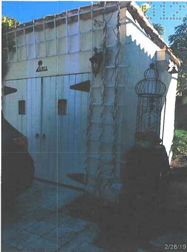
CODE ENFORCEMENT PHOTOGRAPH 6913 TALAVERA STREET
