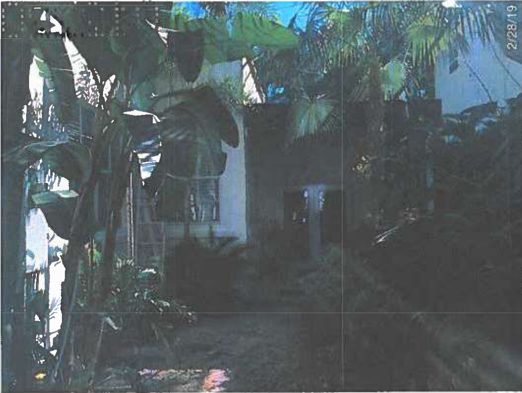
CODE ENFORCEMENT PHOTOGRAPH 6913 TALAVERA STREET
