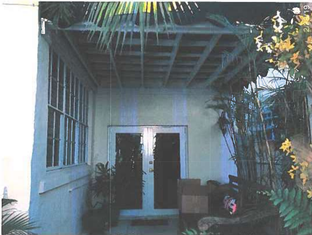
CODE ENFORCEMENT PHOTOGRAPH 6913 TALAVERA STREET
