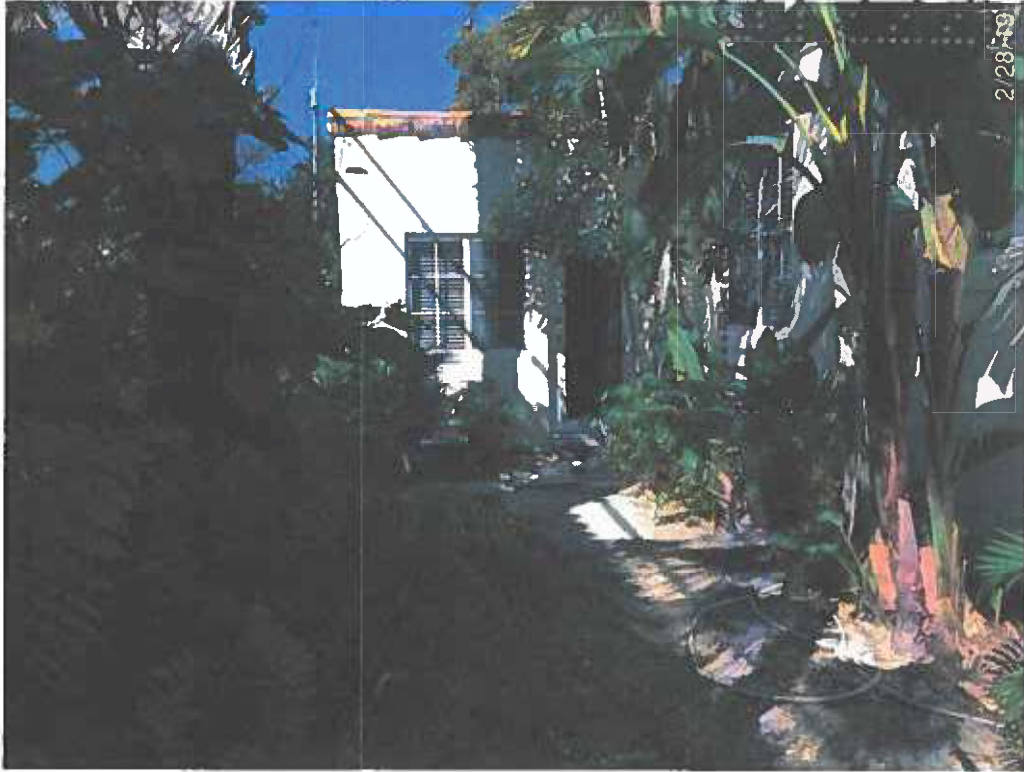
CODE ENFORCEMENT PHOTOGRAPH 6913 TALAVERA STREET
