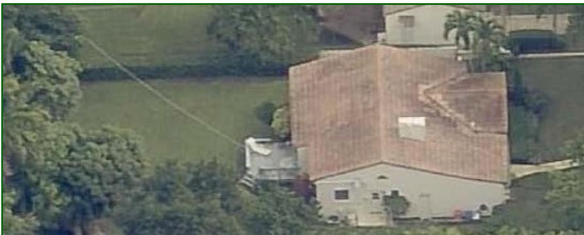
Figures 16: Aerial Photos, 2023 East Façade [top]; Rear (North) Façade [center]; West Façade [bottom]
