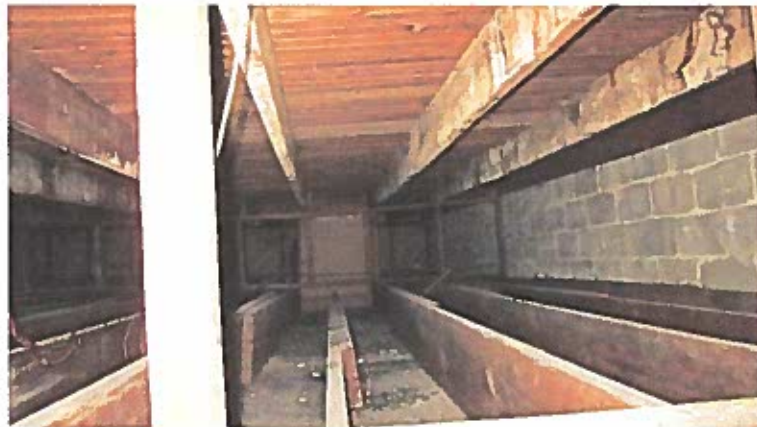
Photograph #8 of wood structure at second floor roof.
