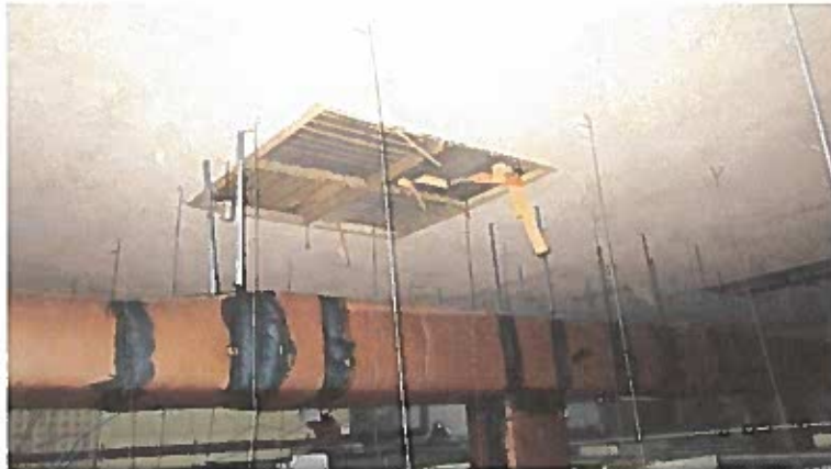
Photograph #6 of underside of concrete slab over main meeting hall first floor roof south wall.
