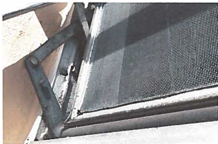
Photograph #9 of aluminum awning window in Legion Hall south wall.
