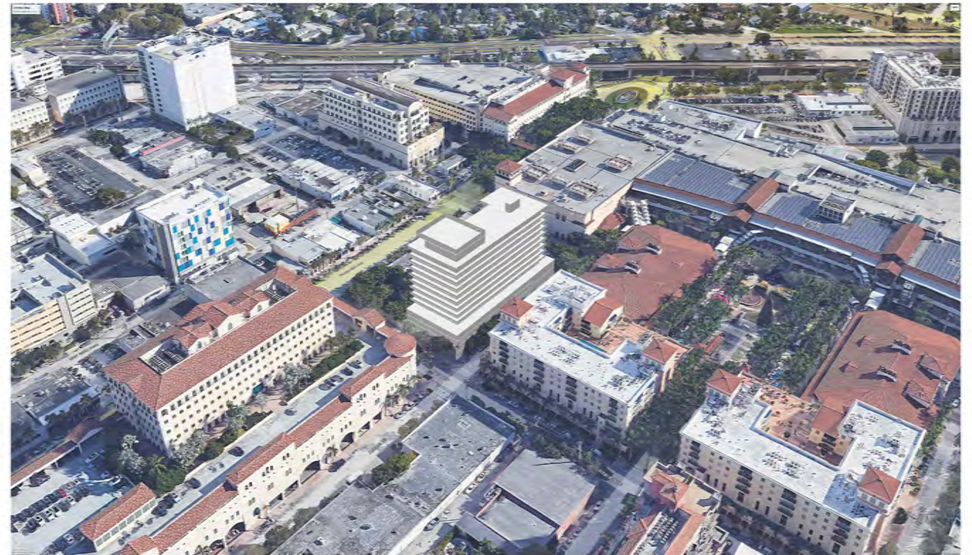
AERIAL LOOKING SOUTHEAST
