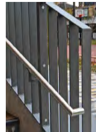
FLAT BAR HANDRAIL
