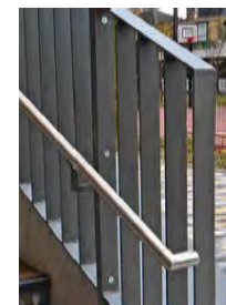
FLAT BAR HANDRAIL
