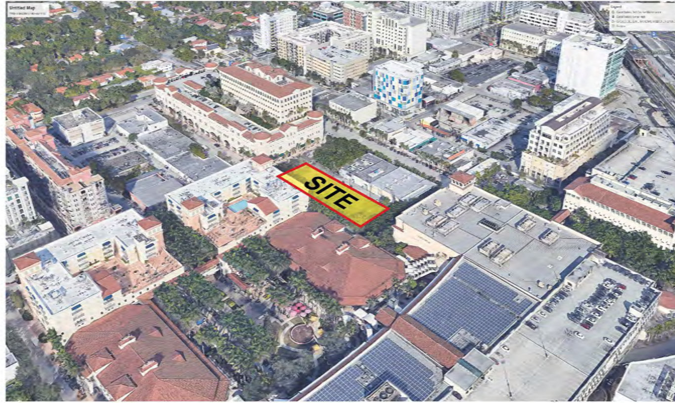
AERIAL LOOKING NORTHEAST
