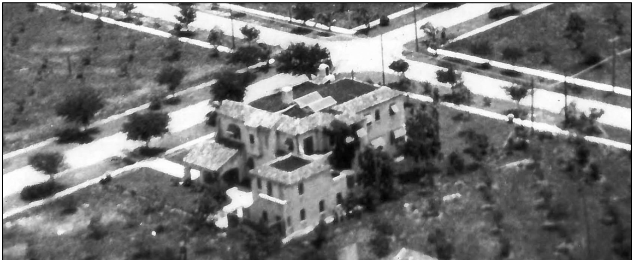
Aerial view from Biltmore Hotel showing rear of 1104 Malaga Avenue, Summer 1930
