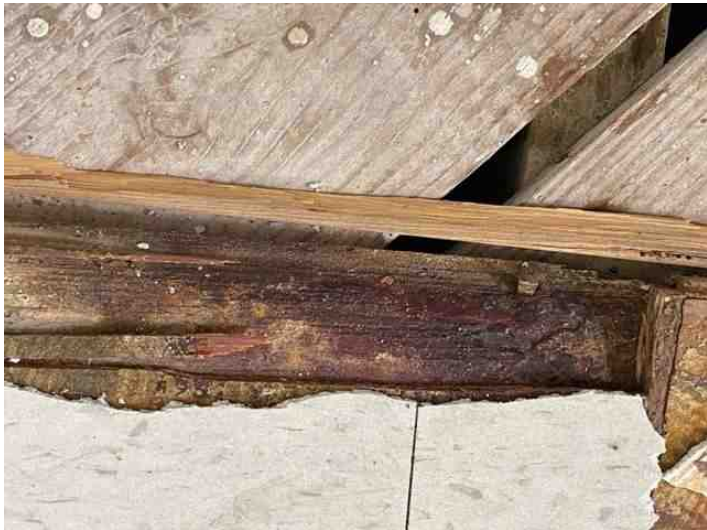
Termite Damage
