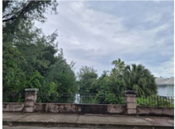
Canal - View north, at the intersection of Pisano Drive and University Drive .
