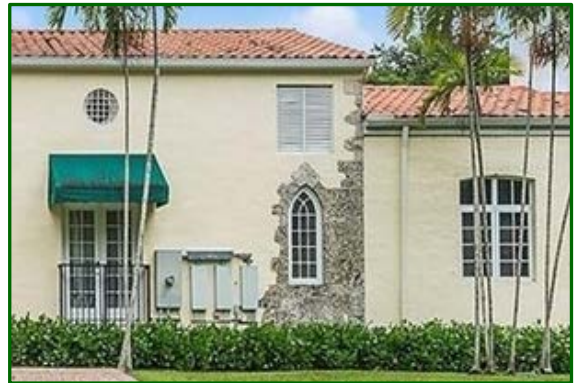
Figure 25: Rear (West) Façade Coral Rock Feature with Gothic Arch Window, 2019
