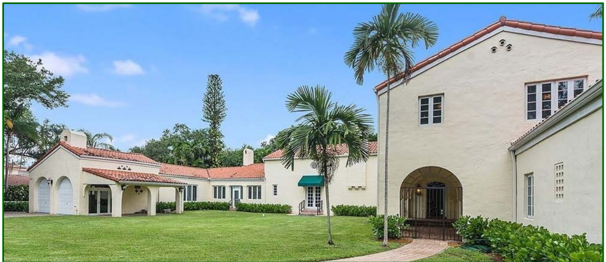
Figures 20: Front Facades Facing Granada Boulevard Northern Wing, South Facades, 2022 [top] Center, East Façade, 2022 [center] Southern Wing, North and East Facades, 2019 Courtesy of Realtor.com [bottom]
