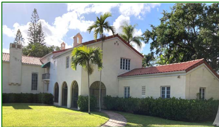
Figure 16: Front Façades looking Northwest, 2022
