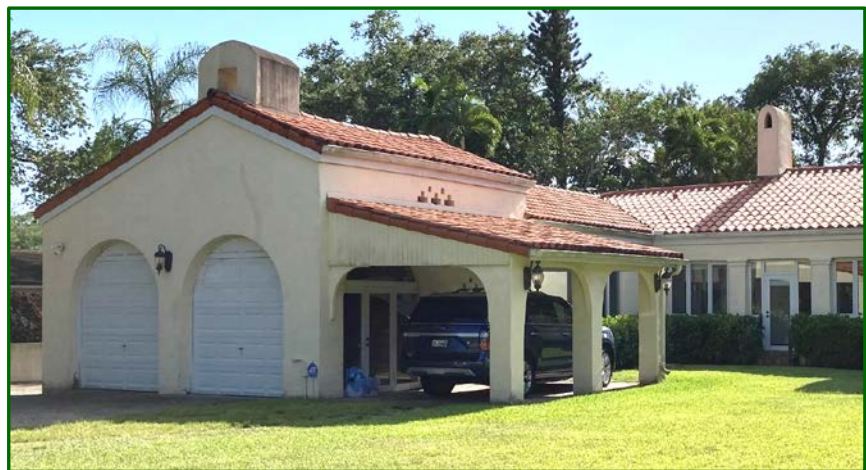
Figure 22: Garage & Carport Bay, 2022
