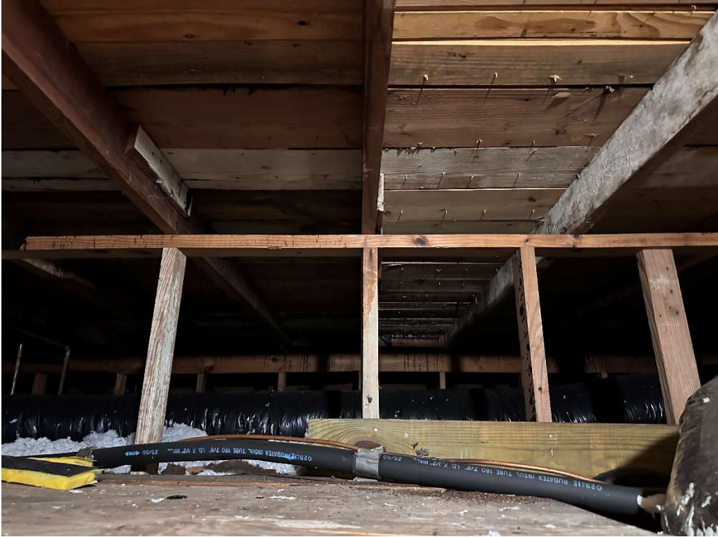
Figure 20 - Wood framing in attic (Section 11b)
