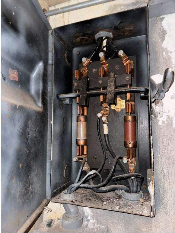
Figure 6 - Grounding of Service (Photo 9)
