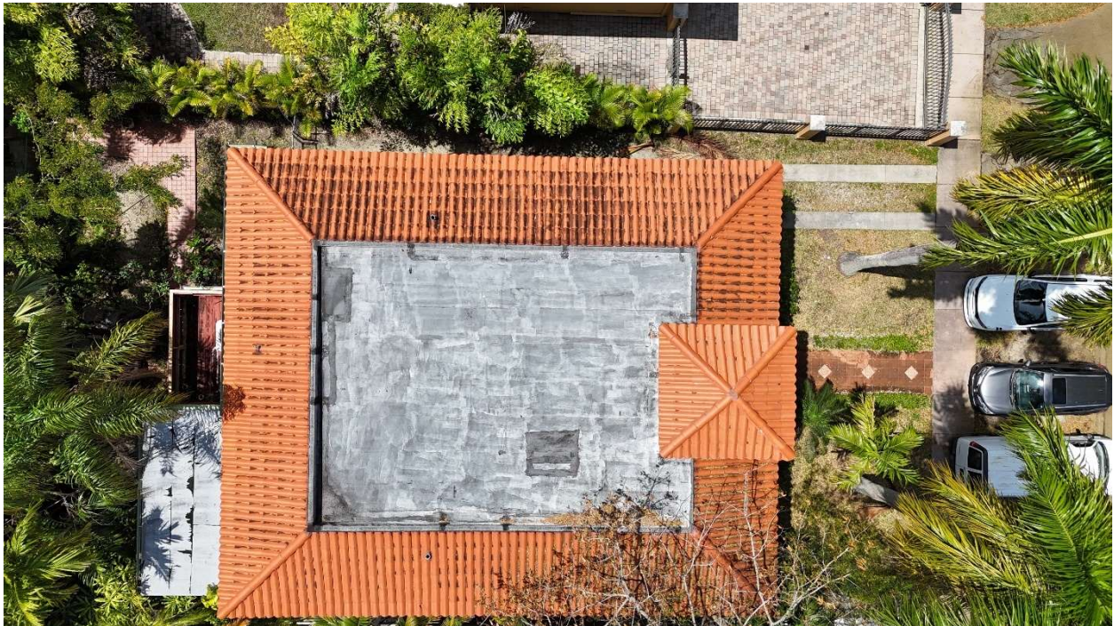
Figure 9 - Roof (Section 7.a.1.)
