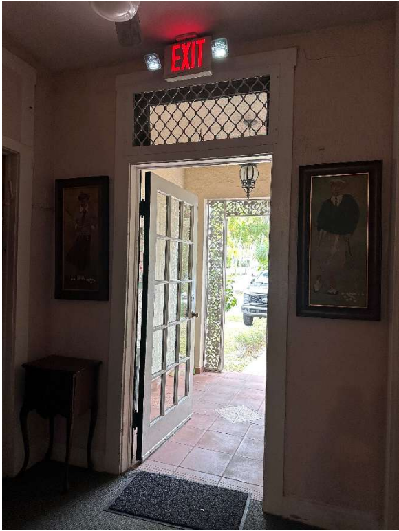
Figure 18 - Exterior door - front door (Photo 10C)
