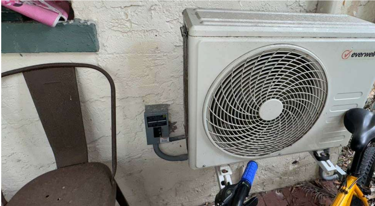
Figure 13 - Wiring to mechanical equipment (Photo 27)
