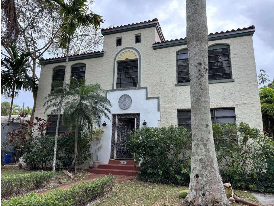
Figure 4 - Present Condition of Overall Structure (Section 5.a.)
