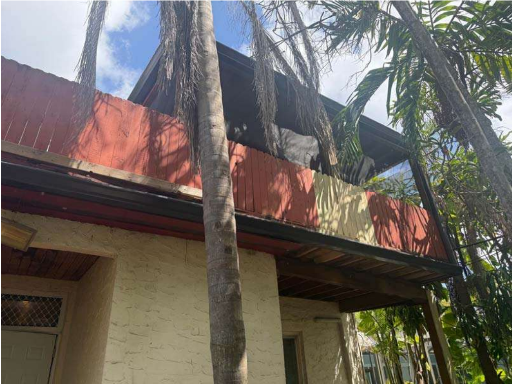
Figure 13 - Balcony (Section 7.b.2)
