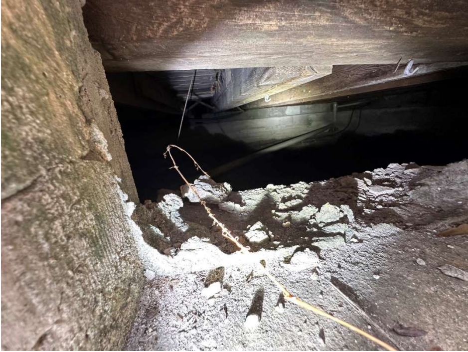
Figure 16 - Concrete Framing (CBS Block) (Section 9.a.)
