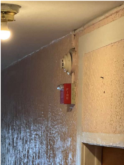
Figure 11 - Existing smoke detectors (Photo 21)
