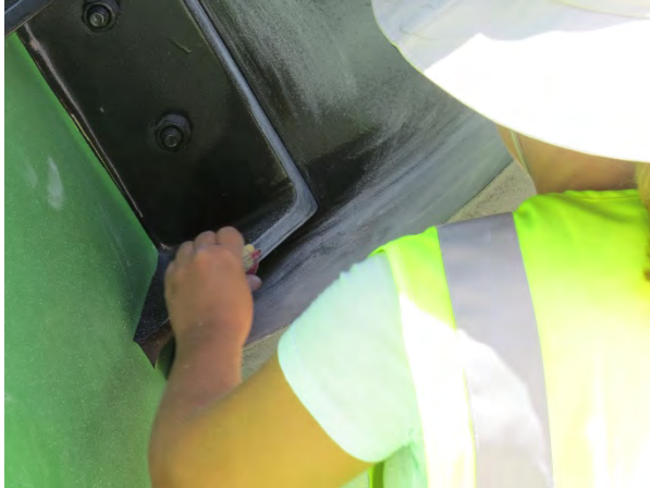
Sanding by hand (left) and with a rotary sander (right), using 80-grit sandpaper.
