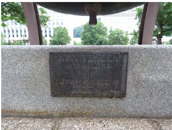
(Left) Tarnishing and corrosion of bronze plate. Note abrasive linear iron staining below the plate. (Right) Loss of gold paint on steel frame and bolts, with localized corrosion. Note blistering of lacquer coating on plaque and corrosion of bronze bell below.
