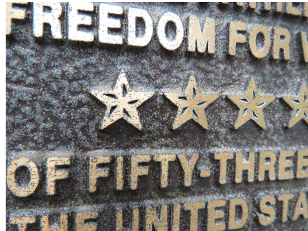
(Left) Linear abrasions with a silvery appearance on the south side of the bell. (Right) Weathered lacquer coating on the dedication plaque.
