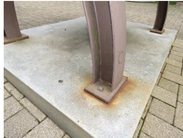
Iron staining on the bell (left) and granite base (right) due to corrosion of iron components. (Right) Note biological growth on the the painted steel leg at the forefront.
