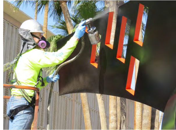
Protecting the surfaces with polyethylene sheeting (left) prior to repainting the black components (right).
