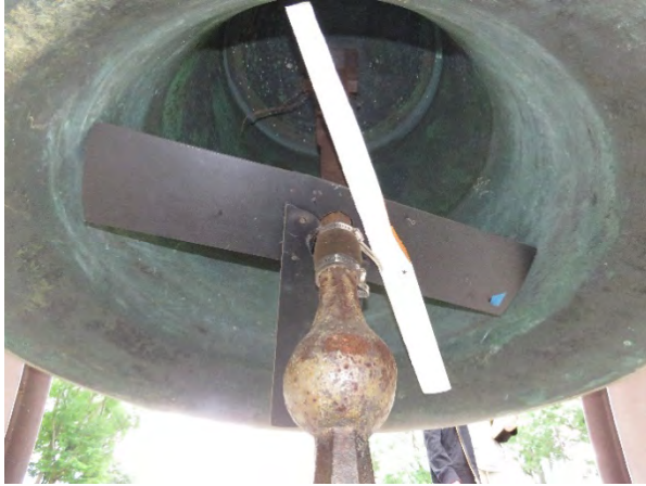
(Left) Corroded clapper held in place with scrap wood and plastic bracing to prevent ringing of the bell. Note corrosion on the interior. (Right) Isolated islands of corrosion around the letters, indicating areas of preferential weathering.
