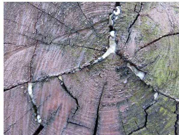
(Left) Sagging and decaying wood yoke, with faded staining. (Right) Biological and possible fungal growths on the ends of the yoke.
