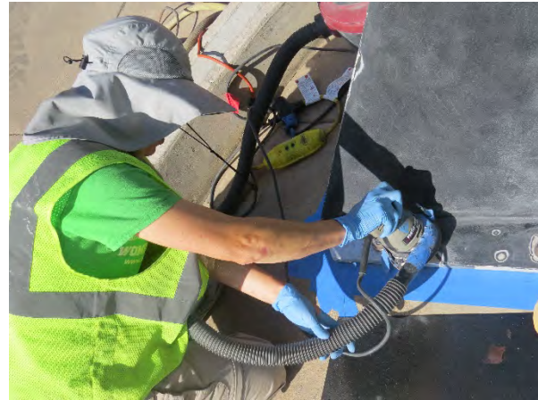
Sanding by hand (left) and with a rotary sander (right), using 80-grit sandpaper.
