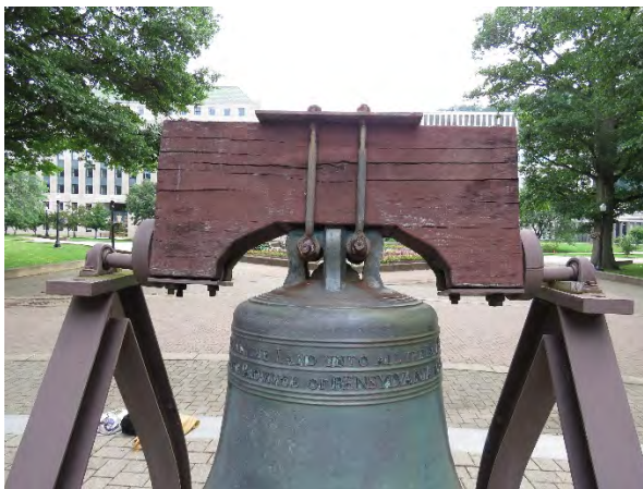
(Left) Sagging and decaying wood yoke, with faded staining. (Right) Biological and possible fungal growths on the ends of the yoke.
