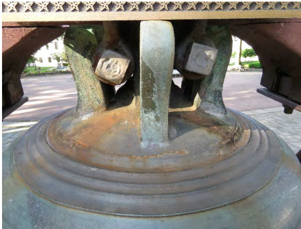
Iron staining on the bell (left) and granite base (right) due to corrosion of iron components. (Right) Note biological growth on the the painted steel leg at the forefront.
