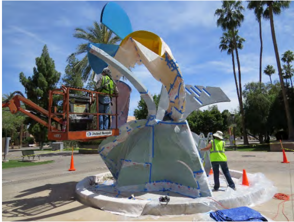
Protecting the surfaces with polyethylene sheeting (left) prior to repainting the black components (right).
