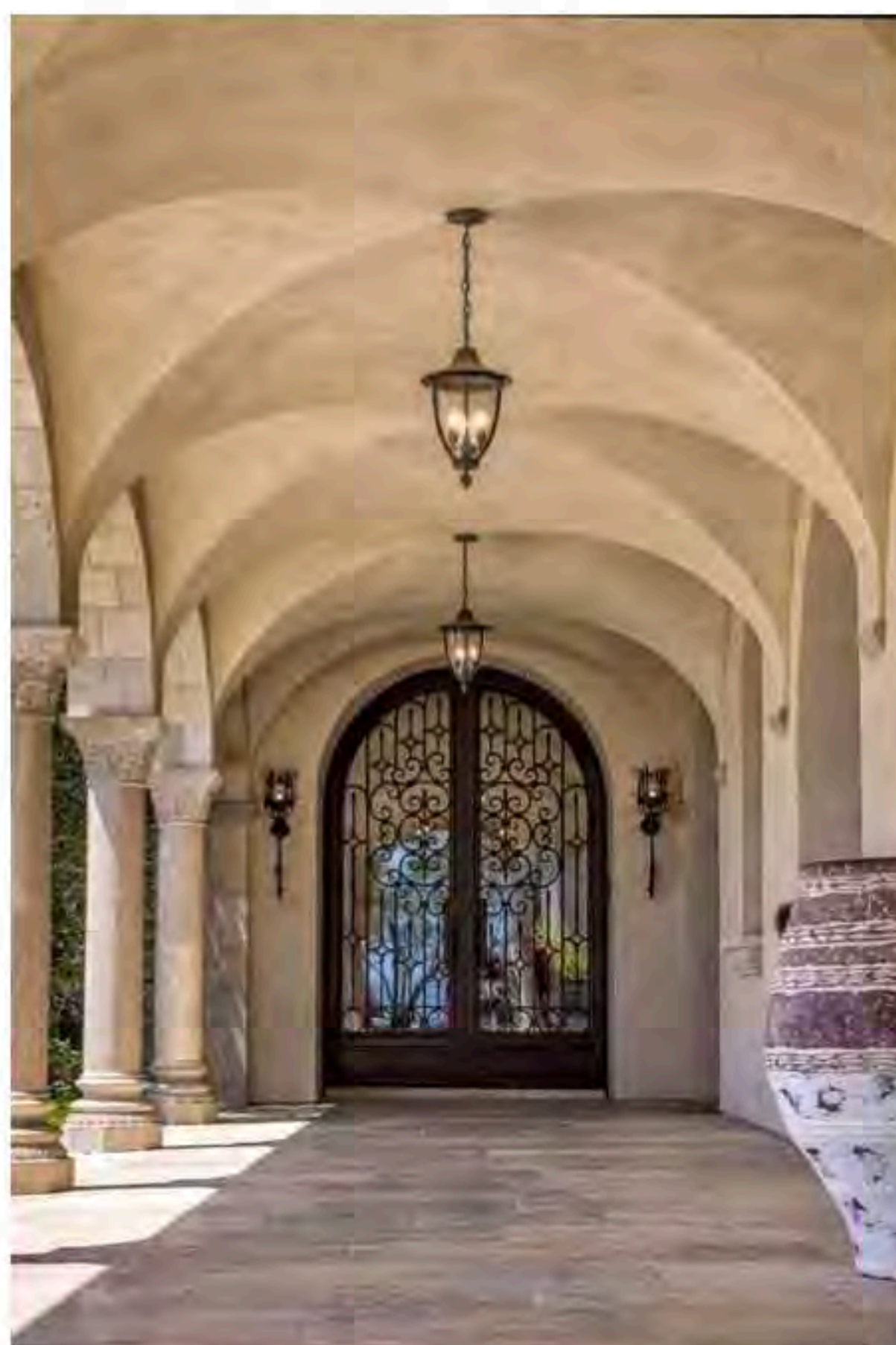
CLASSIC GROIN VAULT INSPIRATION
