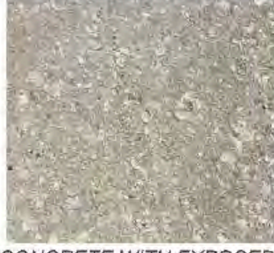
CONCRETE WITH EXPOSED COQUINA SHELL AGGREGATE
