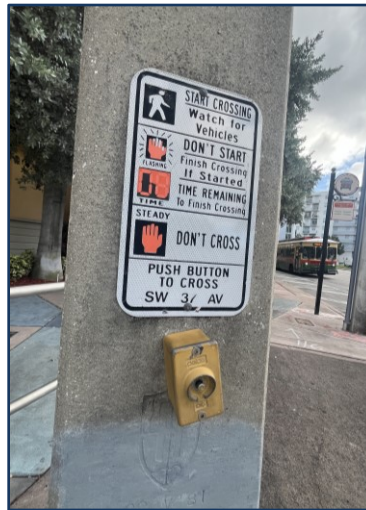
Photo 4: Pushbutton tilted and Sign faded (NE corner)
