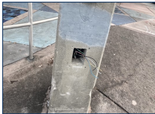
Photo 5: Exposed Wires (Upright NE Corner)
