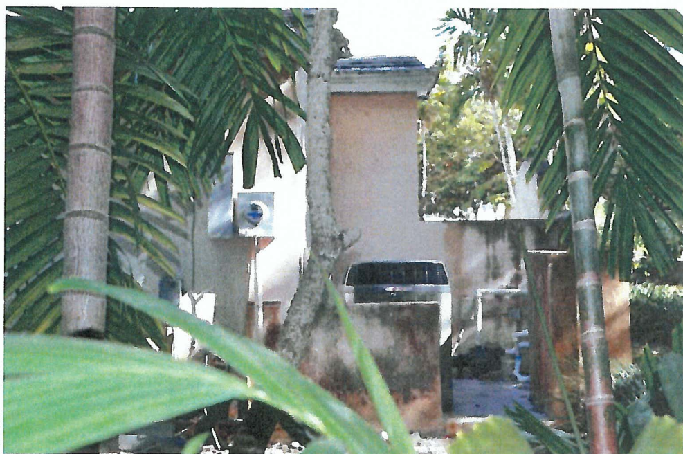
Adjacent View of Home East of New Construction
