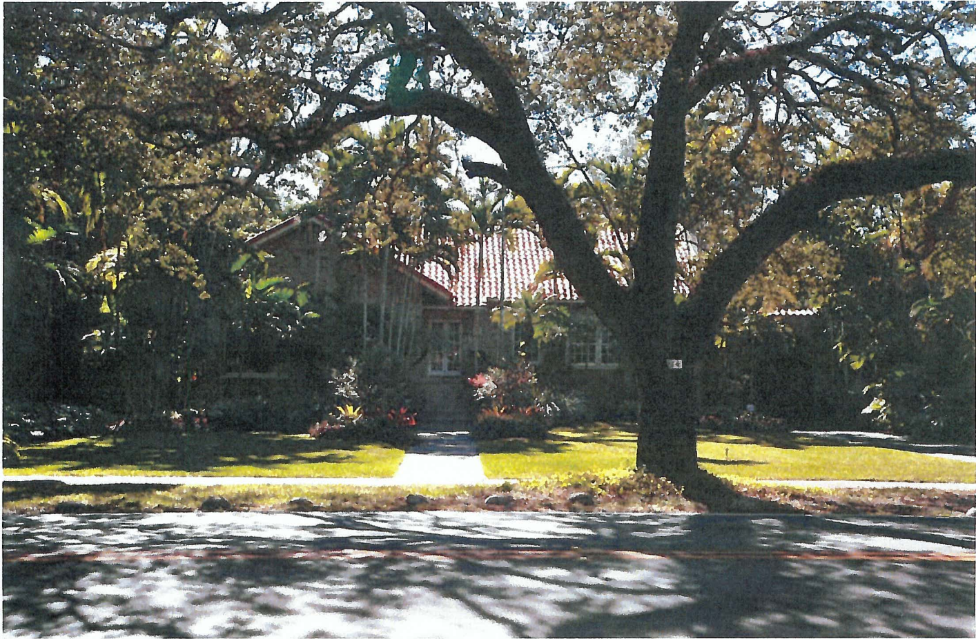
Existing House (North Façade)
