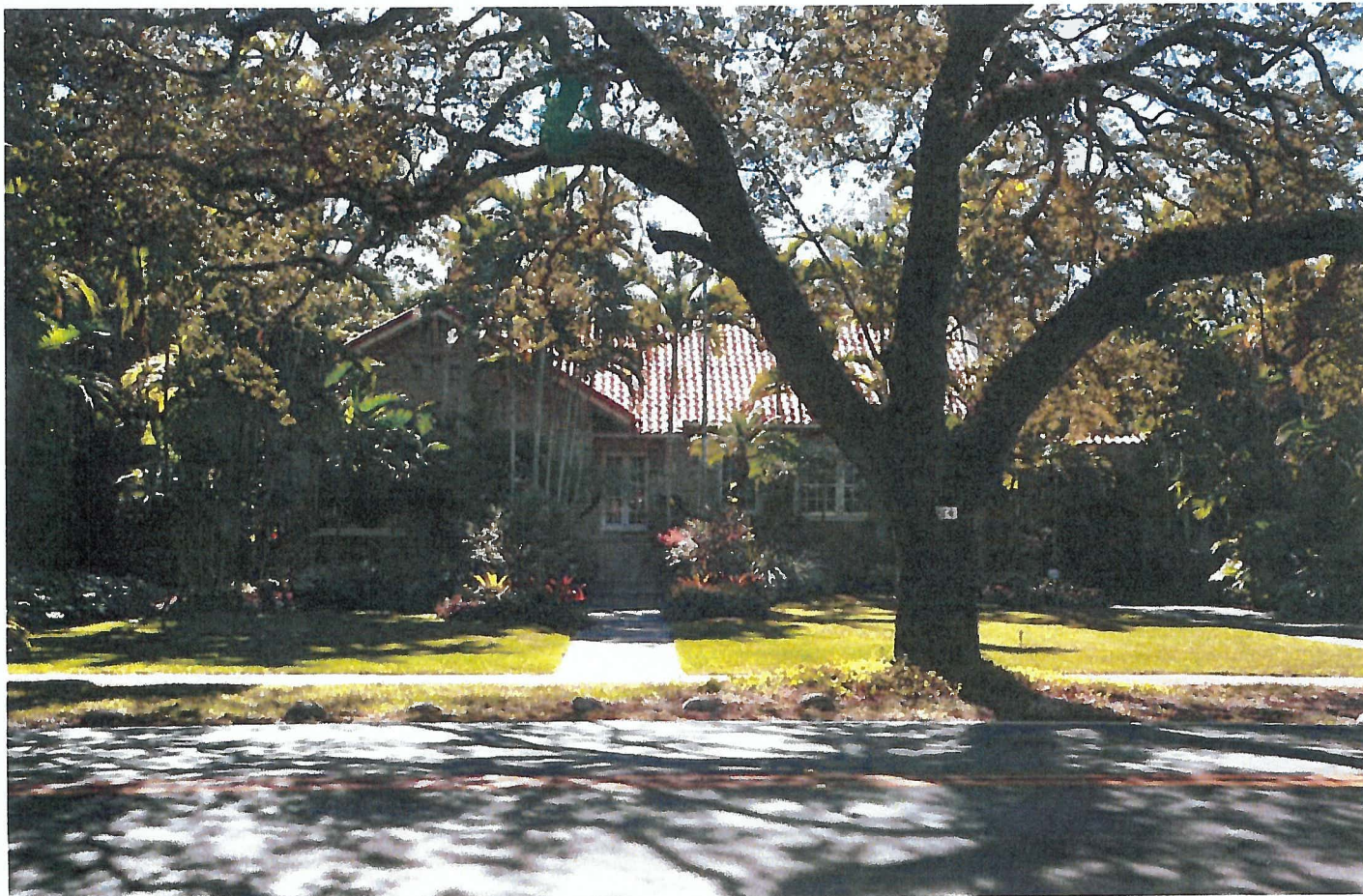
Existing House (North Façade)
