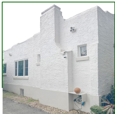
Figure 19: West Side Façade: Chimney, 2025
