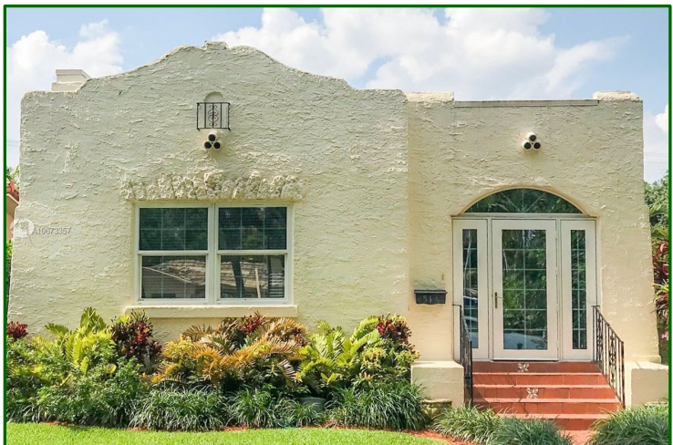
Figure 16: Front (South) Façade 2025 [top]; 2019 [bottom]
