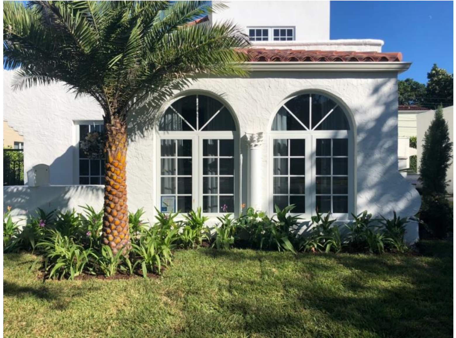
West (Front) Façade – Porch After
