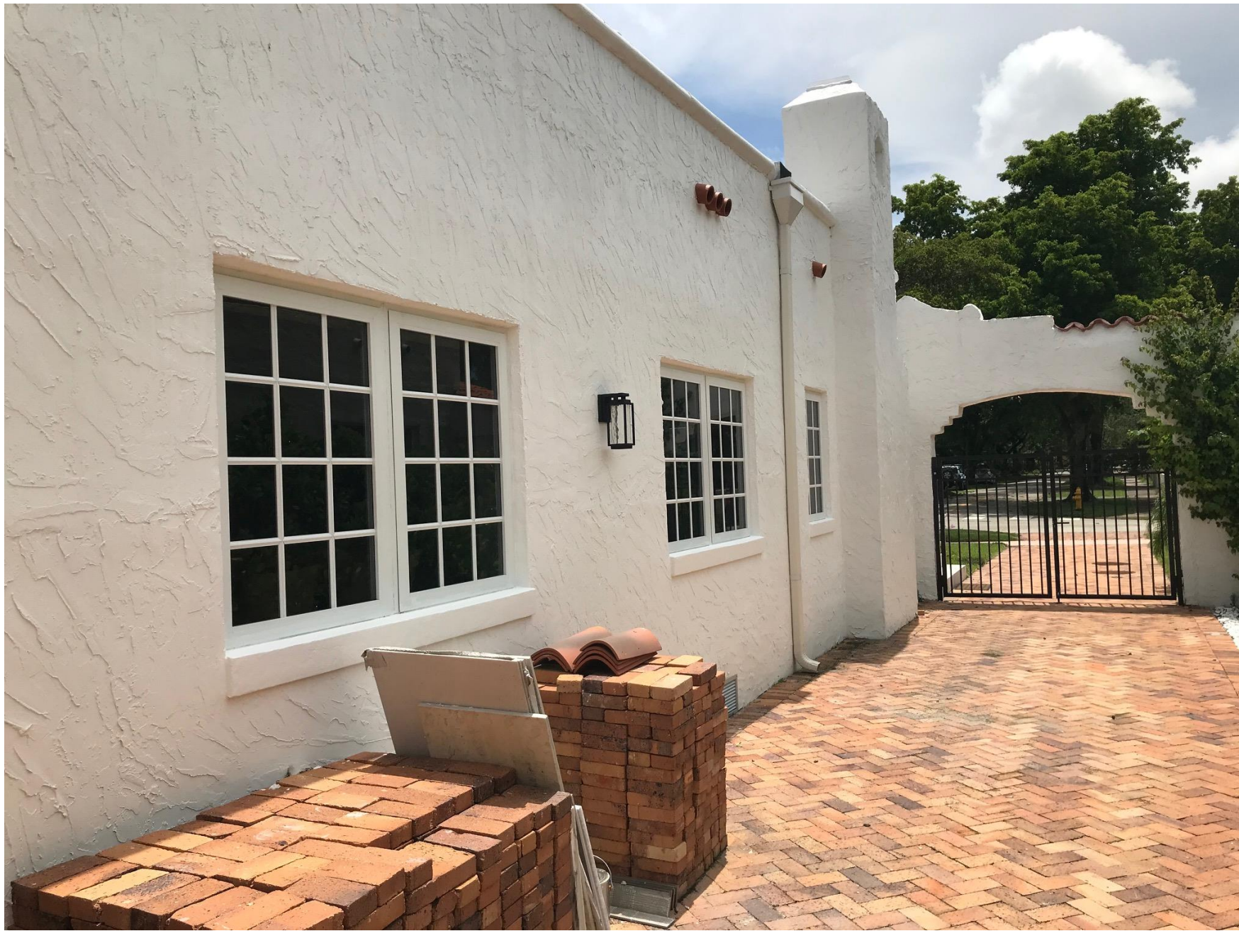
North Façade –After
