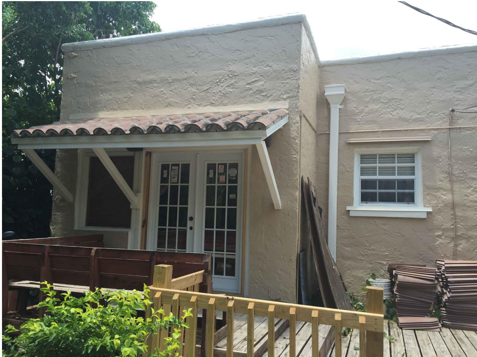
East (Rear) Façade – Before
