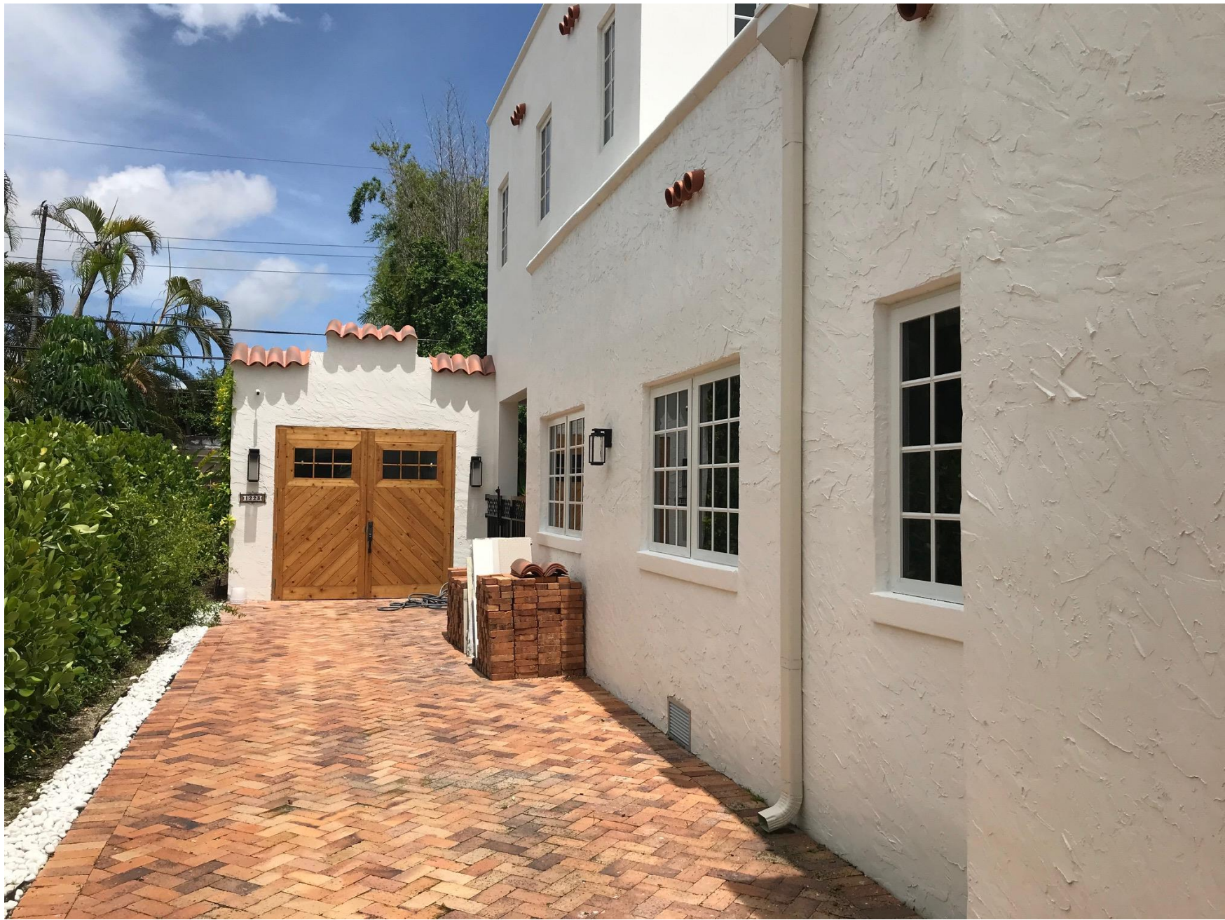
North Façade –After
