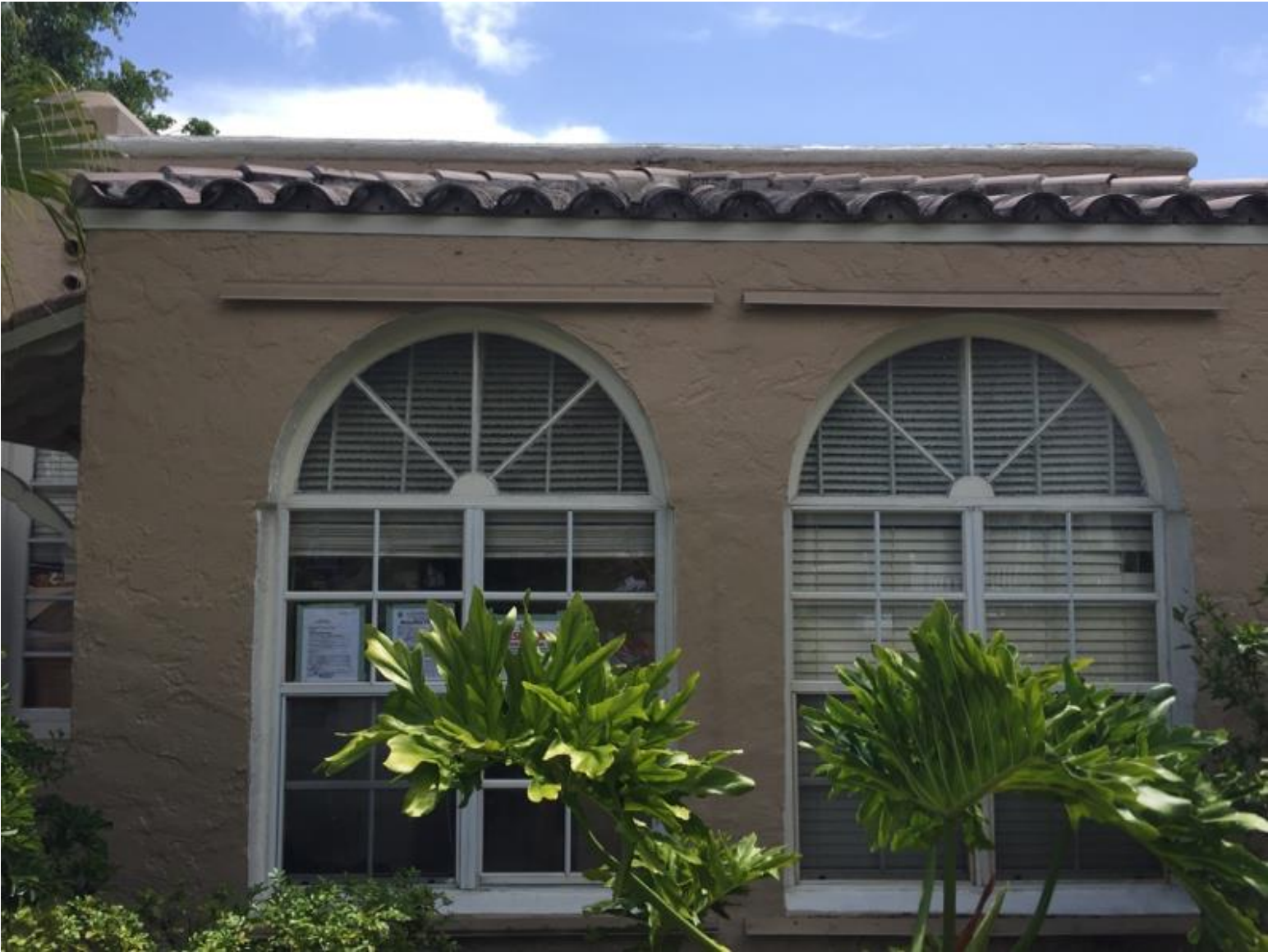
West (Front) Façade – Porch Before
