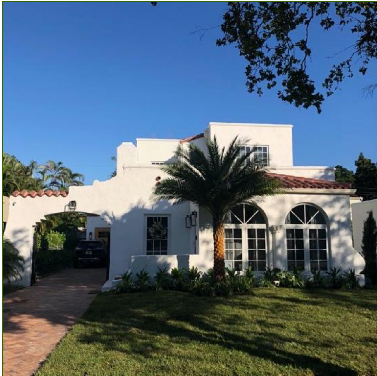
North (Front) Façade - After
