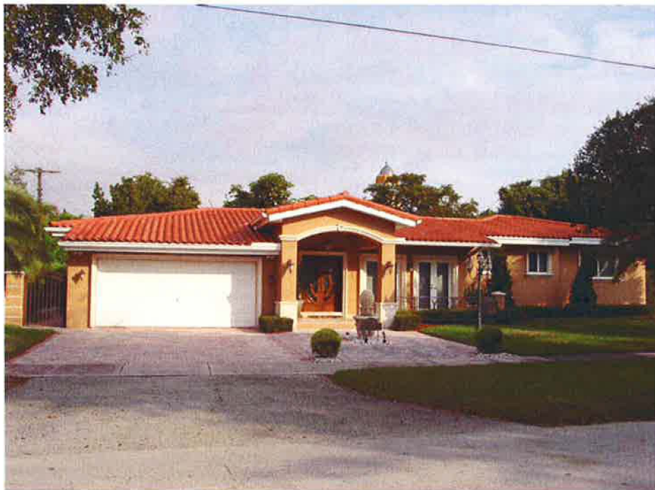
1501 South Greenway Drive – 2007
