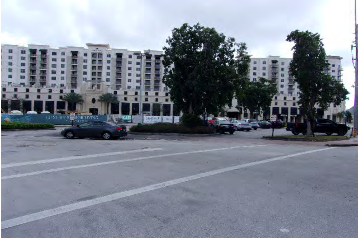
LOOKING SOUTHEASTERLY AT SUBJECT FROM GRECO AVENUE
