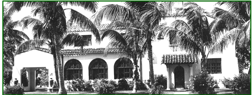
Figures 26: Front (East) Façade: Note Differences 1925 Permit #1160 [top]; Post-1947 Historic Photo [bottom]
