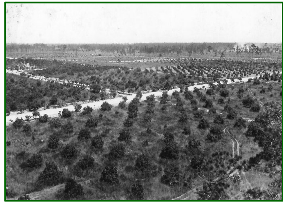
Figure 2: Streets in Coral Gables under Construction, July 22, 1922
