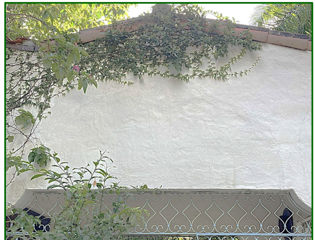
Figure 27: Porte Cochere, West Façade, 2026 Note: Semicircular Outline Visible in Stucco
