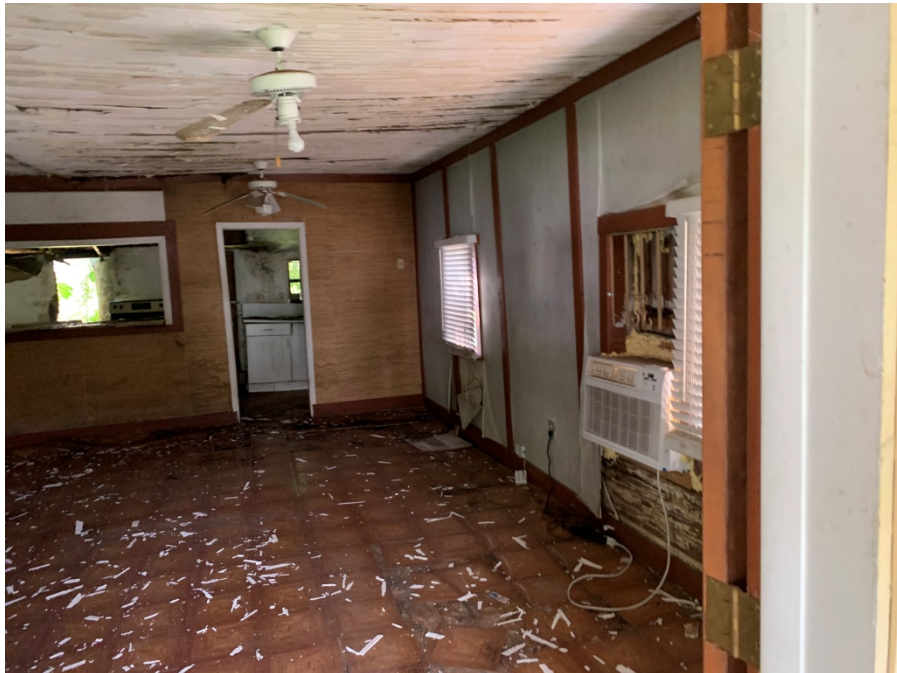
Picture #6 Interior of the house
