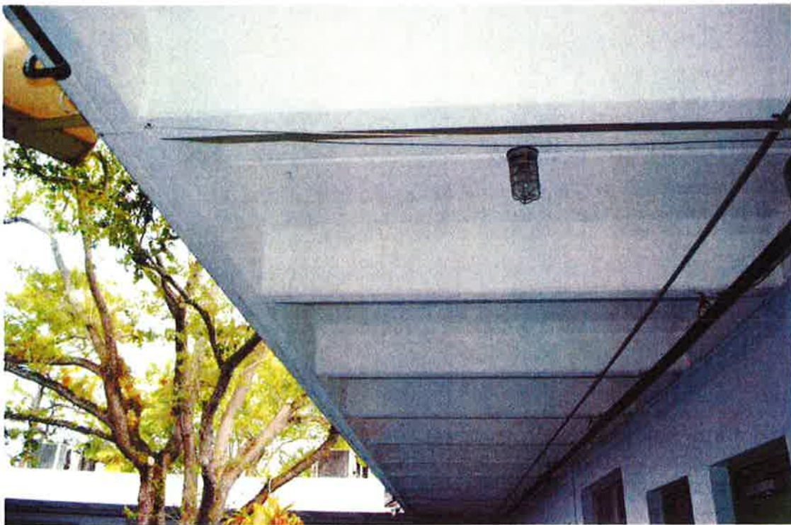
Figure 5: Typical Exposed Beam Ceiling Detail within Walkways Surrounding School Courtyard
