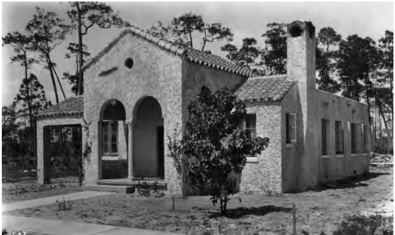
Southeast Elevation (House in the 1920's)
