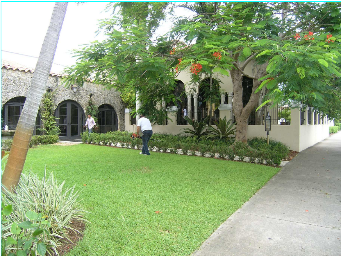
GREENWAY ENTRANCE LOOKING EAST
