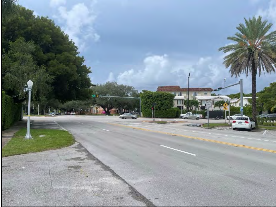
Le Jeune Road at University Drive, East Leg (Facing West): No residual queues after green time ends.
