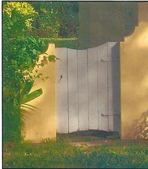
Figure 11: Detail of Wing Wall and Gate, Front (South) Elevation, December 2016
