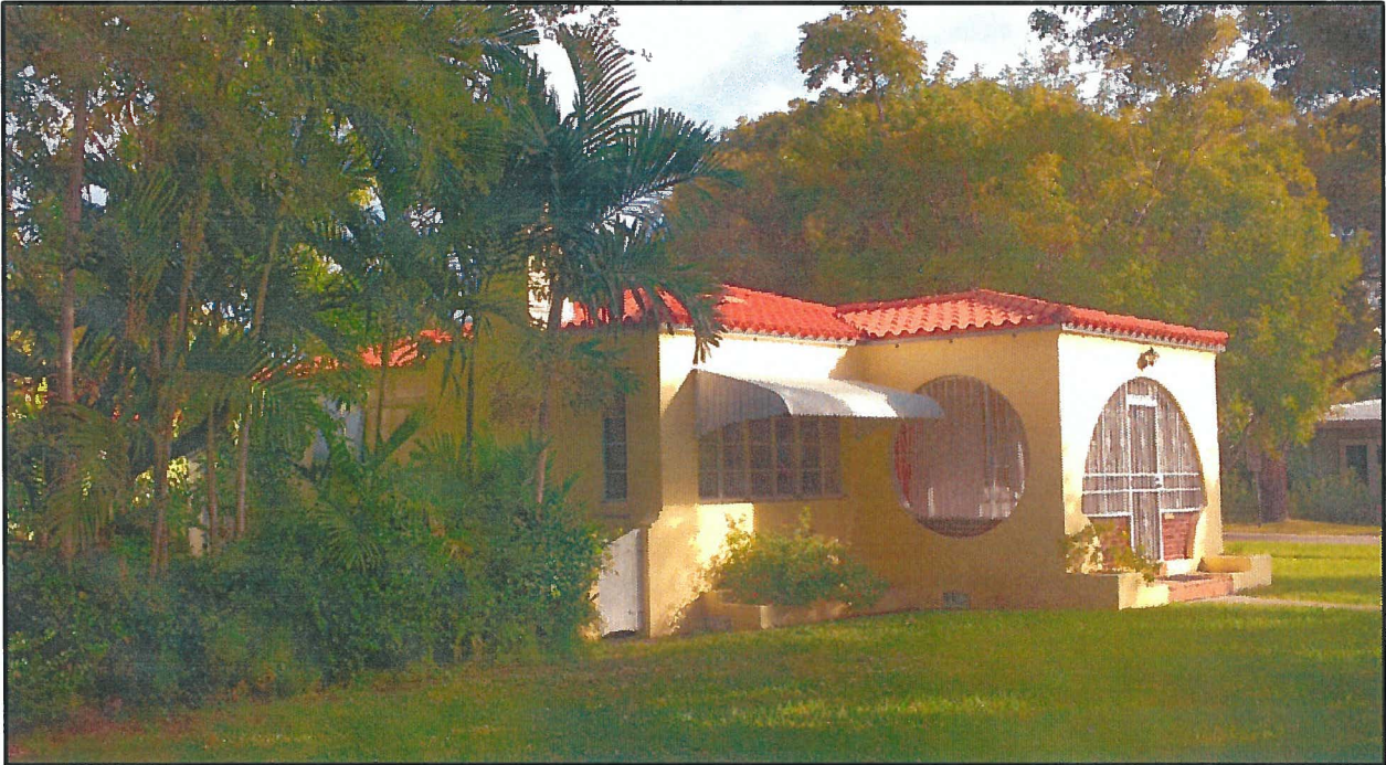
Front Elevation (South) Looking Northeast
