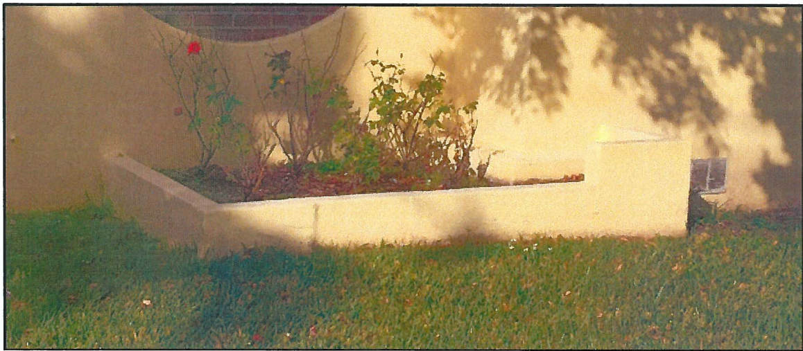
Figure 9: Built-in Planter Detail at East side of Entry Porch, December 2016
