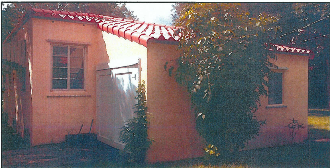
Figure 14: Rear (North) Elevation, October 2016 Photograph submitted with Historic Significance Request
