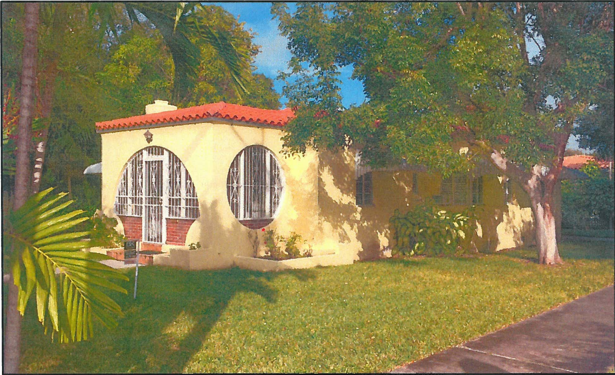
Front Elevation (South) Looking Southwest
