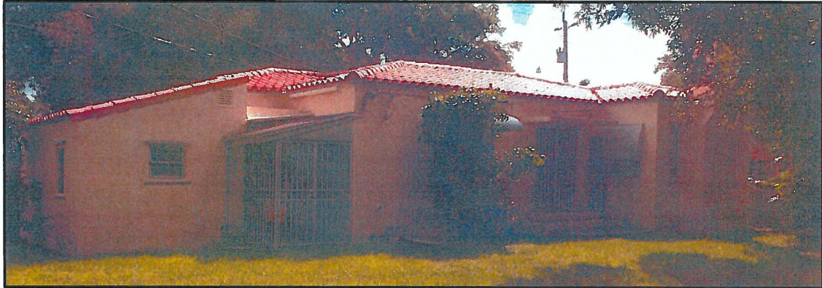
Figure 15: West Elevation, October 2016 Photograph submitted with Historic Significance Request
