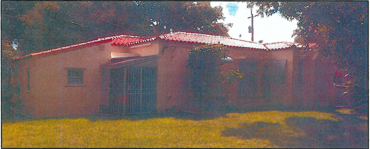
Side Elevation (West) - Photograph Submitted with Historic Significance Request
