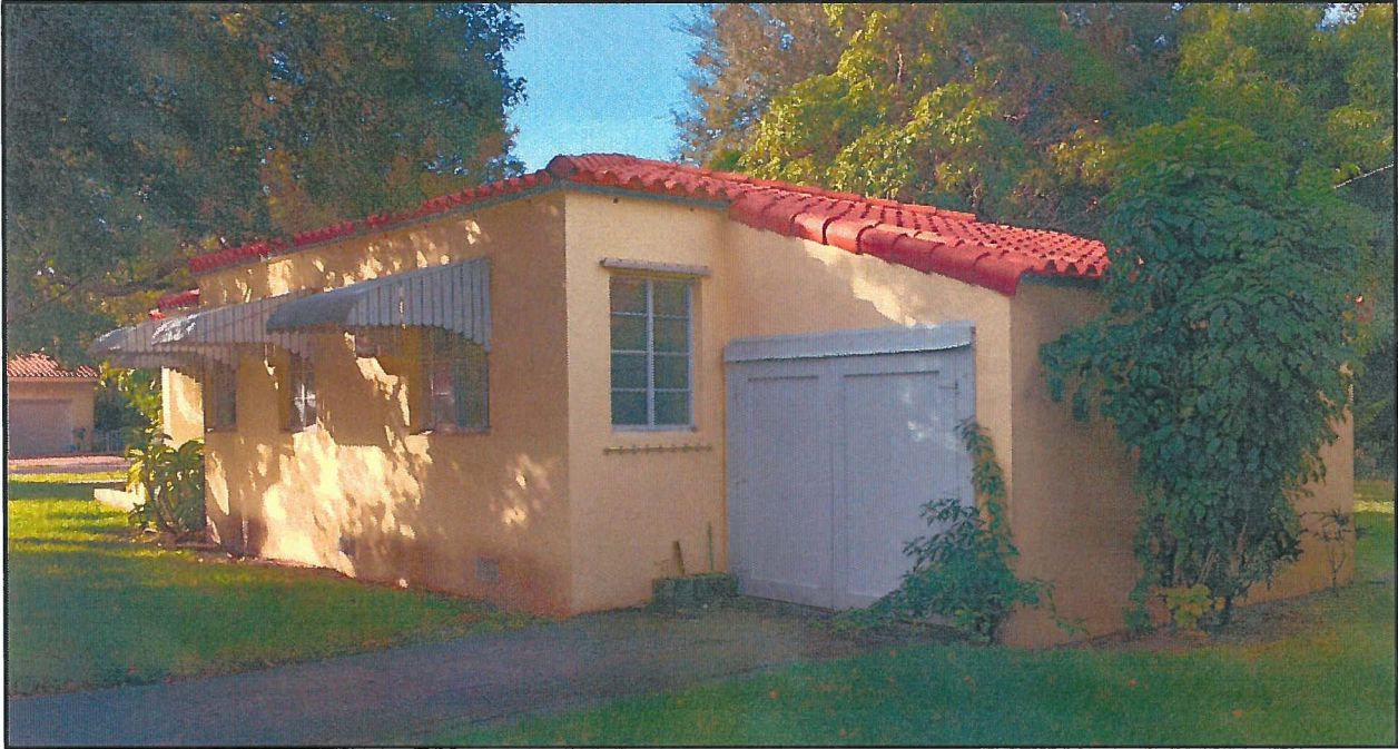
Side Elevation (East) Looking Southwest
