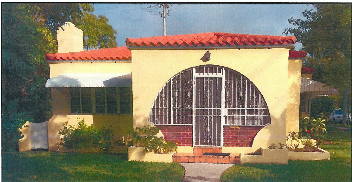
Figure 8: Front (South) Elevation, December 2016
