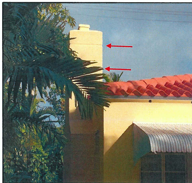
Figure 10: Detail of Chimney, Front (South) Elevation, December 2016
