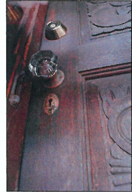
Figure 3: Existing Side Door
