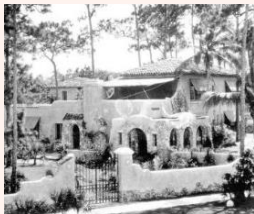
Merrick Mansion (832 South Greenway)
