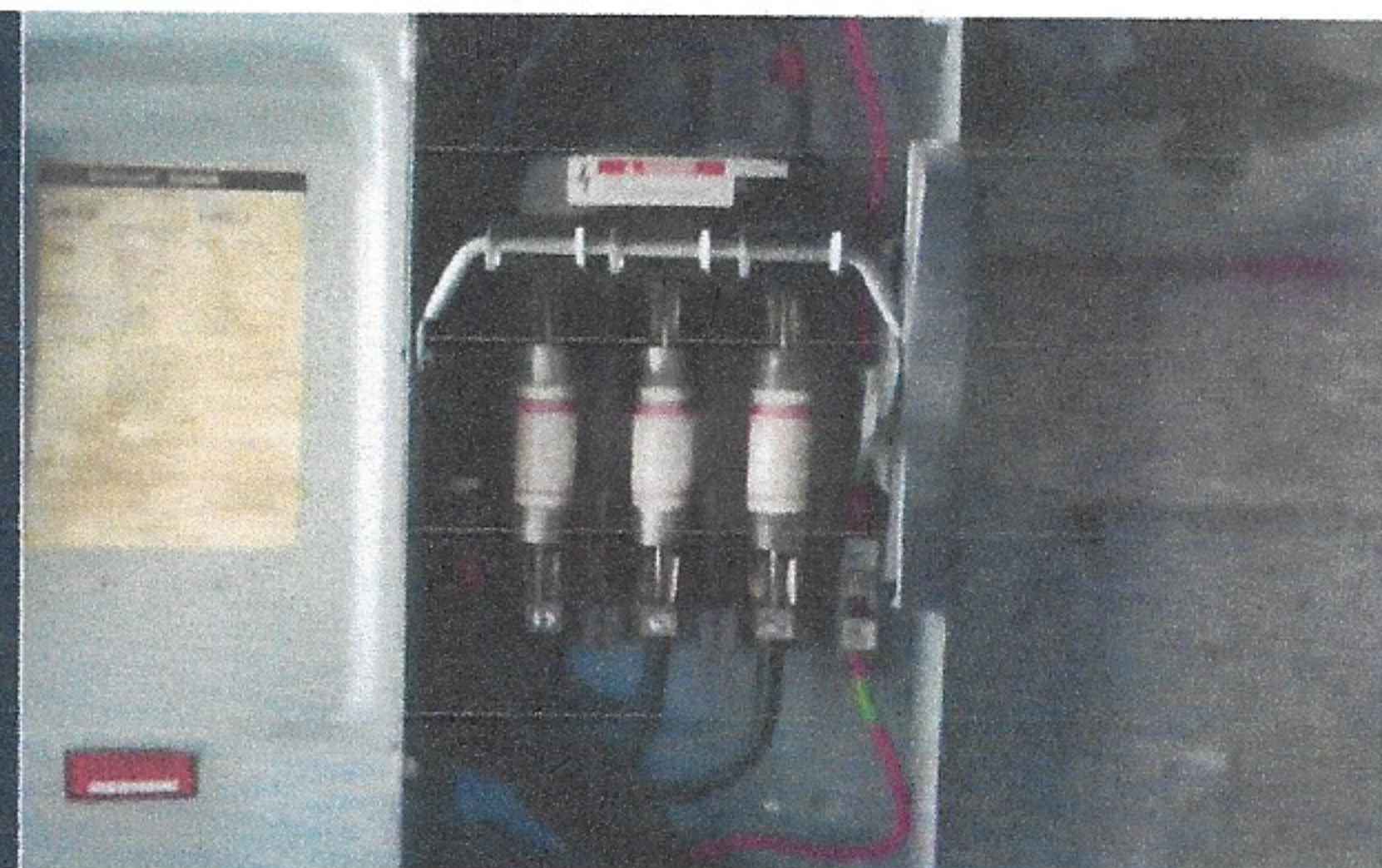
4800 Elevator Sub.jpegAligned Visual Image
