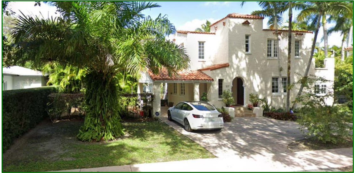
Figure 9: Avenue, Front (South) Façade, 2022 Courtesy of Google Earth
