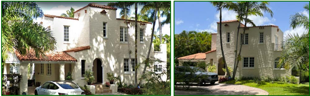
Figures 11: Front (South) Facade, 2022
