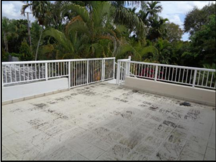
Second Floor Terrace
