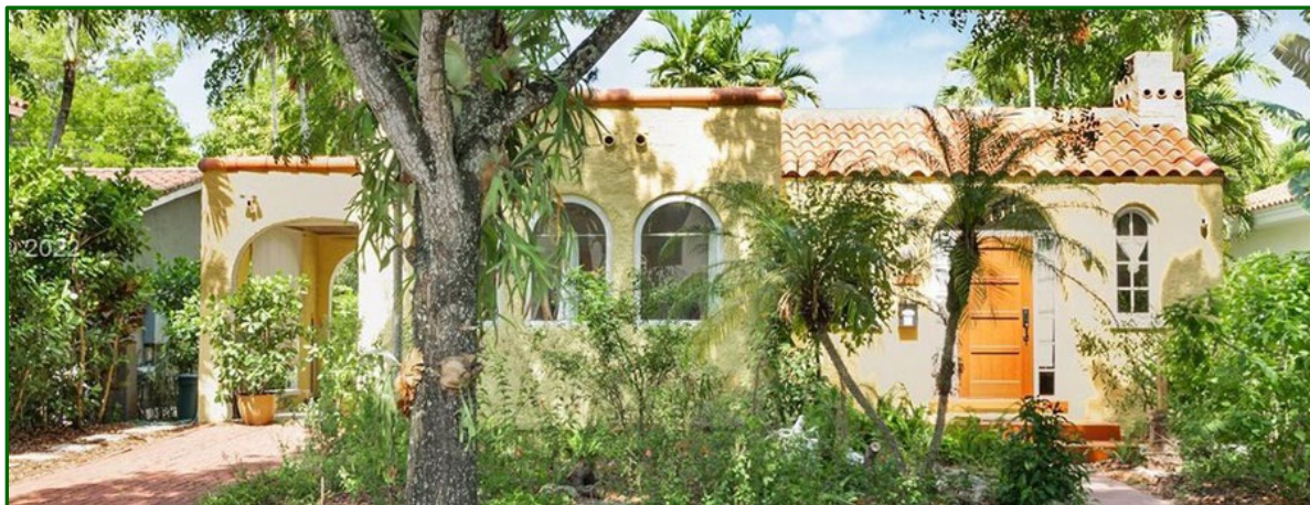
Figures 9: 1116 Alberca Street Overview over Time Permit #1780, 1925 [top]; Historic Photos: c.1940 [center]; Current, 2022 Courtesy Realtor.com [bottom]
