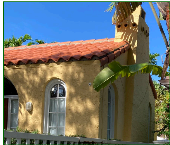
Figure 14: Entry Bay with Chimney, 2024
