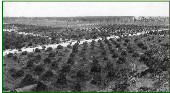
Figure 1: Streets in Coral Gables under Construction, July 22, 1922
