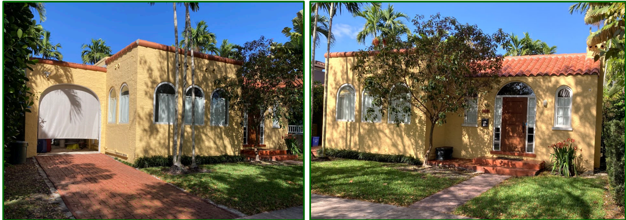
Figures 13: Front (East) Façade, 2024
