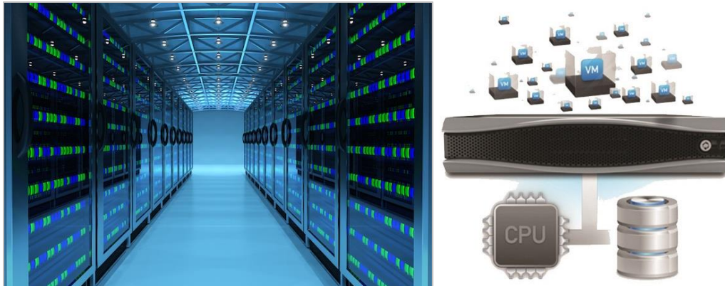
Figure 12. Illustration of datacenter and hyper-converged infrastructures (HCIS) and cloud scalability
