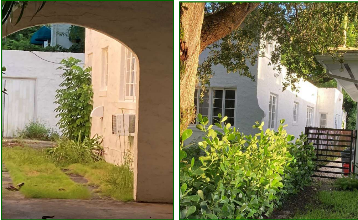
Figures 13: Side Facades, 2021 Looking North: West Façade [left]; East Façade [right]
