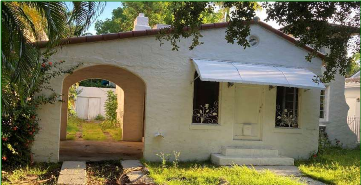
Figures 7: 1129 Sevilla Avenue, Front (South) Facade c.1940s [top]; Current, 2021 [bottom]
