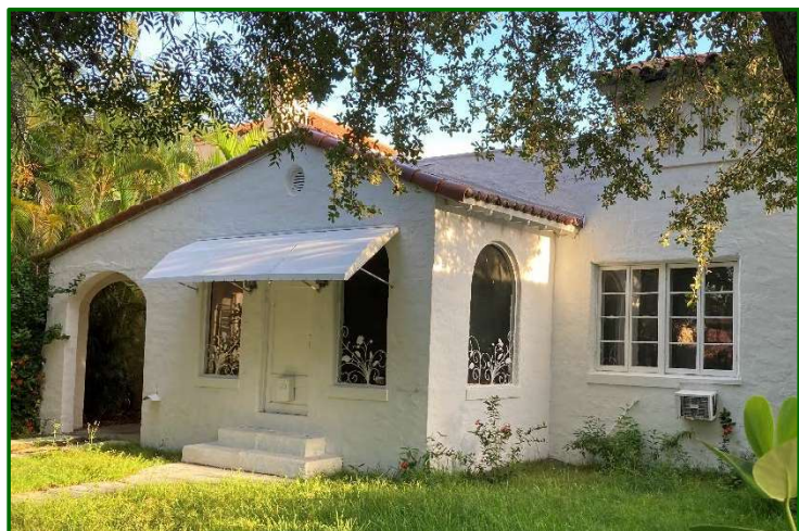
Figure 12: Front Covered entry Porch, looking northwest, 2021
