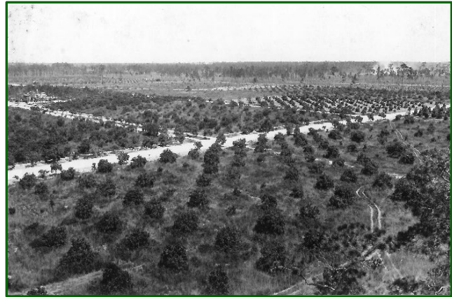
Figure 2: Streets in Coral Gables under Construction, July 22, 1922
