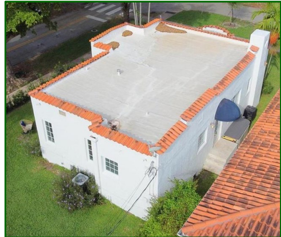
Figure 30: Aerial Photo of Rear (East) & North Side Facades, 2020
