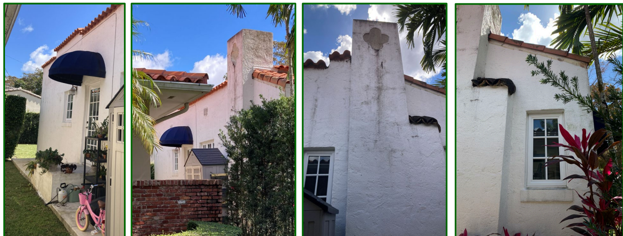
Figures 31: North Side Façade Permit 1330, 1925 [top]; Current Photos, 2026
