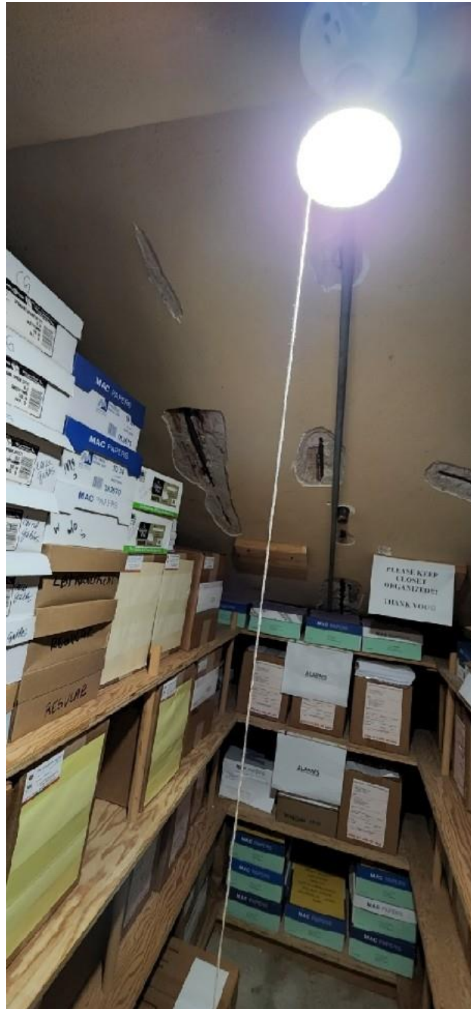
PHOTOGRAPH 5 - SPALLING BELOW MAIN STAIRCASE
