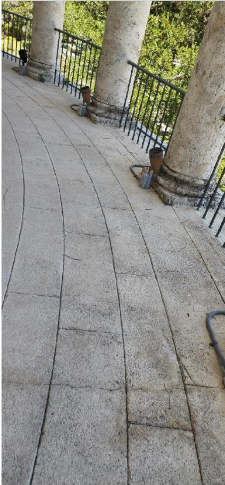
PHOTOGRAPH 33 - LOOSE BALCONY TOP RAILING
