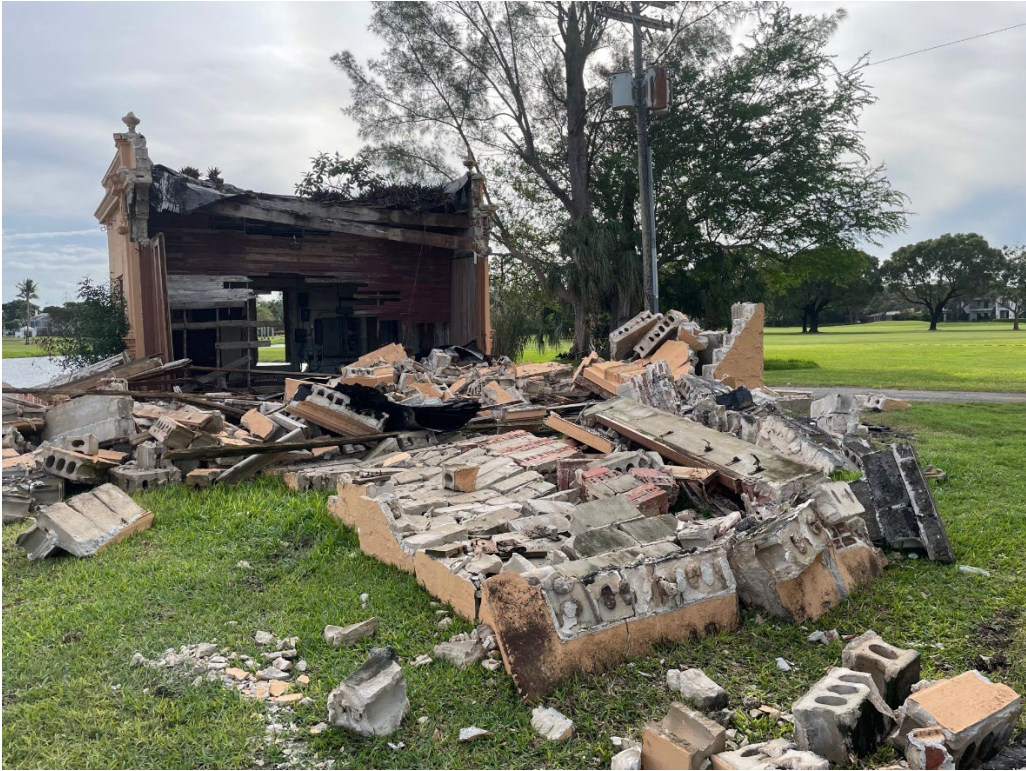
Gondola Building, December 2021
