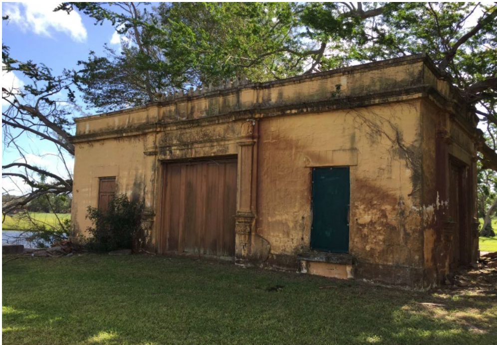
Gondola Building, December 2017
