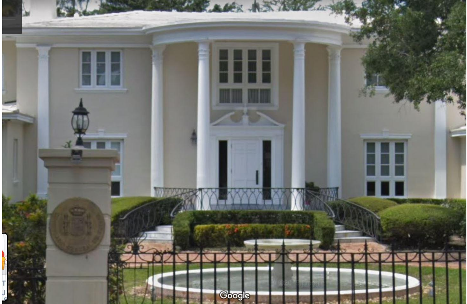
Elaborate Front Doorway with Broken Pediment and Decorative Surrounds at 3600 Granada Blvd
